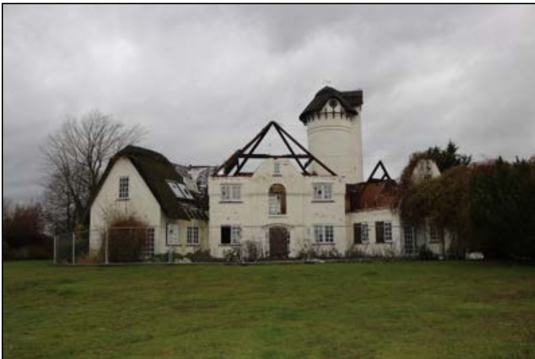
Plate 2 Exterior of the building, from the rear with central south-east range/cow house with wings, taken from the south-east (DP 012)
