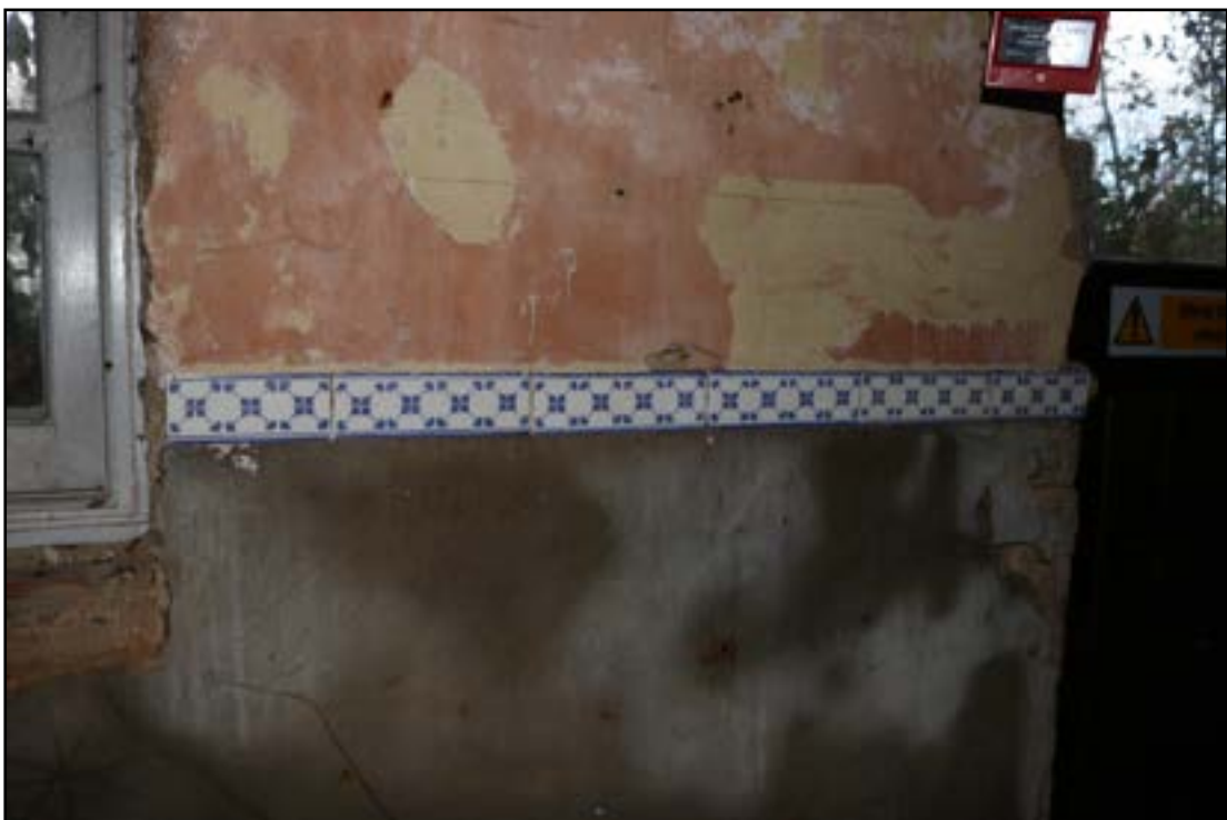
Plate 8 Detail of lower cementitious render divided from gypsum plaster by decorative tile, in the south-west range, taken from the north-east (DP 067)
