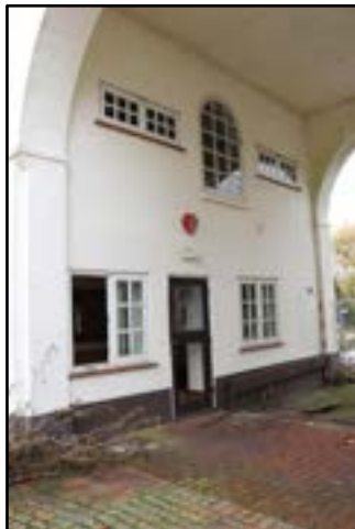
DP 39 West side of the gateway, taken from the south- east
