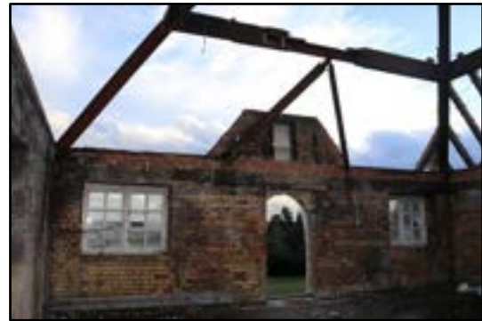
DP 122 Surviving upper structure to the south-east range, taken from the north-east
