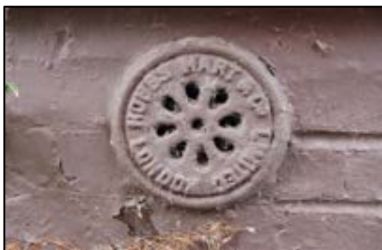
DP 41 A Hobbs, Hart & Co. iron plate to the west side of the gateway, taken from the north-east
