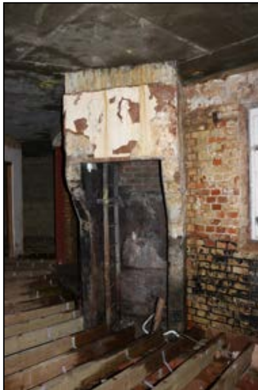
Plate 6 Access ladder for the silo within the north-east arm, taken from the north-east (DP 088)
