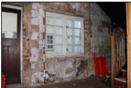
DP 105 Evidence of tiles within the gateway range, taken from the south-east
