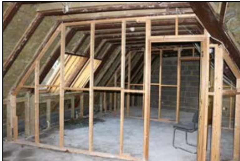
Proposal 1: example of the studwork partitions to be removed (DP 136)
