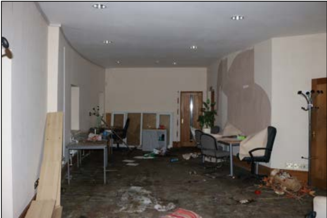
Plate 7 View of the interior of the west wing, taken from the south-east (DP 058)
