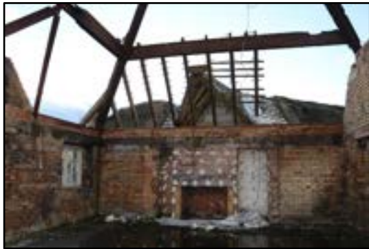
DP 121 Surviving upper structure to the south-east range, taken from the north-east
