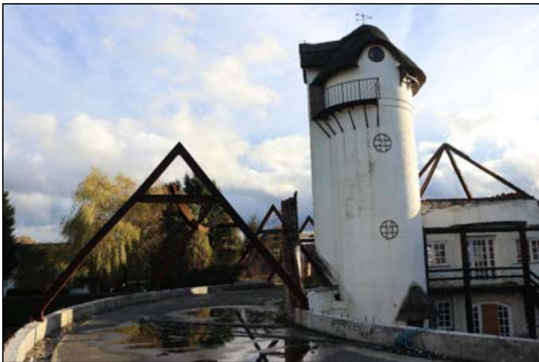
Plate 4 Surviving upper structure above the north-east arm, taken from the east (DP 112)
