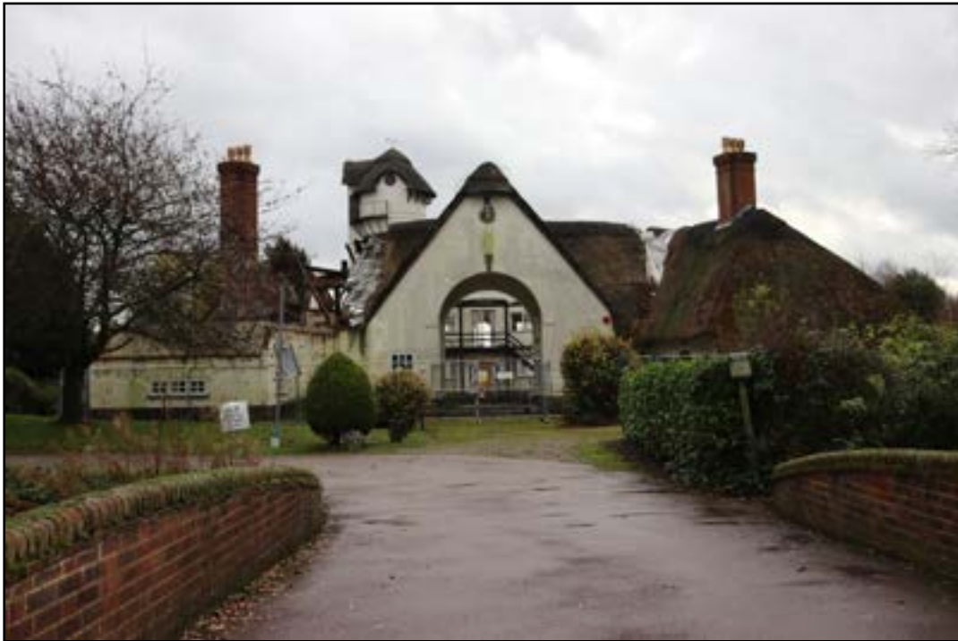
Plate 1 Exterior of the building, from the approach driveway with central gateway range with flanking wings, taken from the north-west (DP 001)
