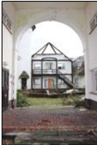
DP 37 View through the gateway, into the courtyard, taken from the north-west
