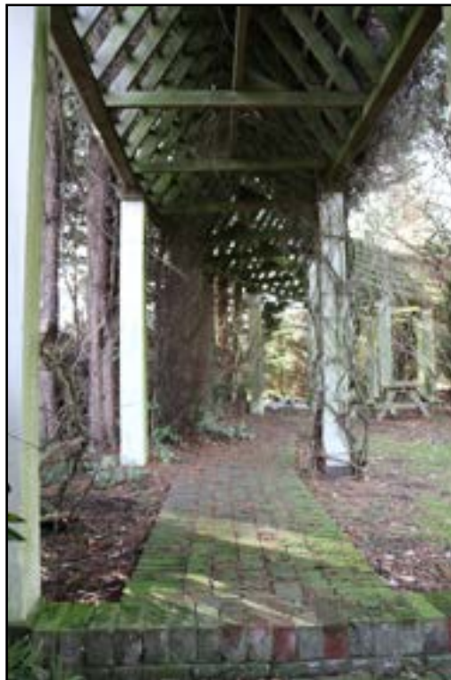
Plate 10 Walkway between the Dairy and the Midden, taken from the south-east (DP 144)
