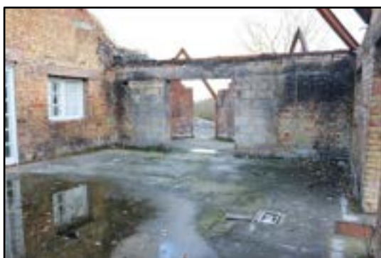
DP 125 Surviving upper structure to the south-east range, taken from the south-west
