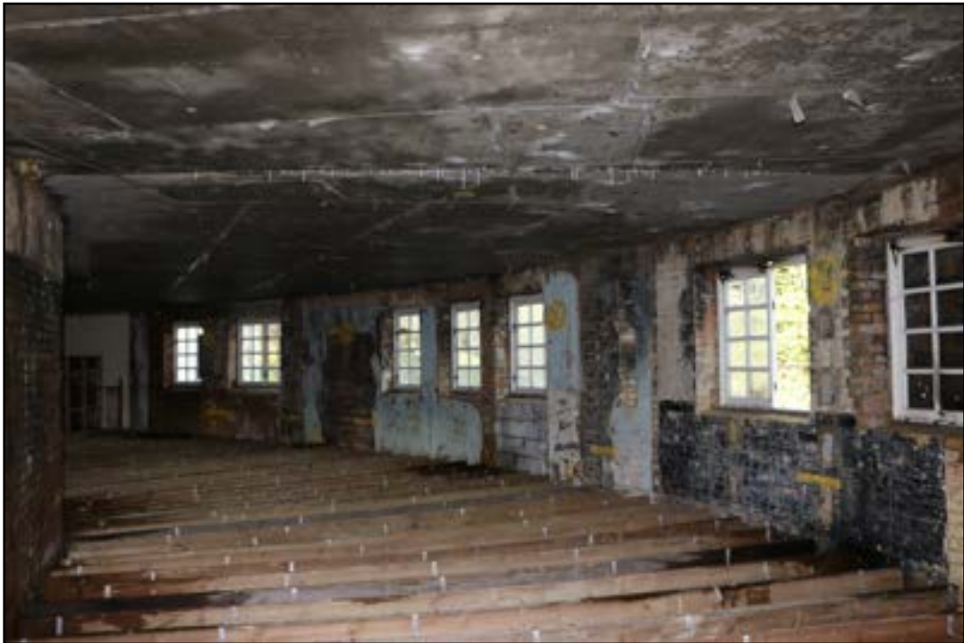
Plate 9 Interior of the north-east arm, showing scarring of previous subdividing walls, taken from the south (DP 091)
