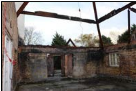
DP 123 Surviving upper structure to the south-east range, taken from the west
