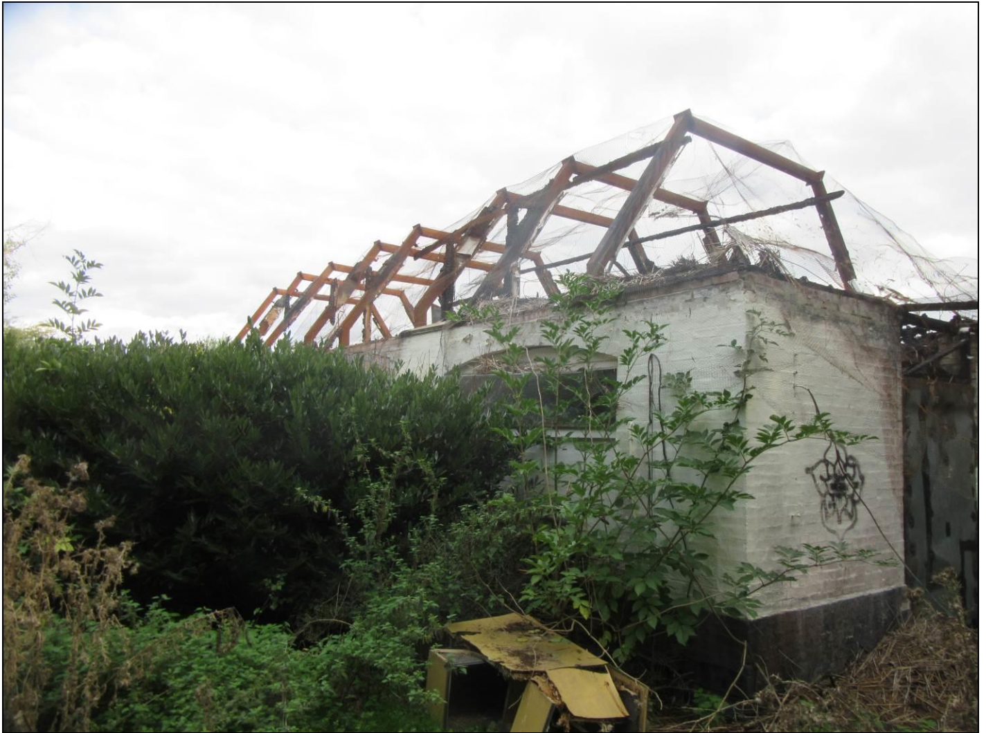
Photograph B – Showing the derelict building to the rear site boundary.
