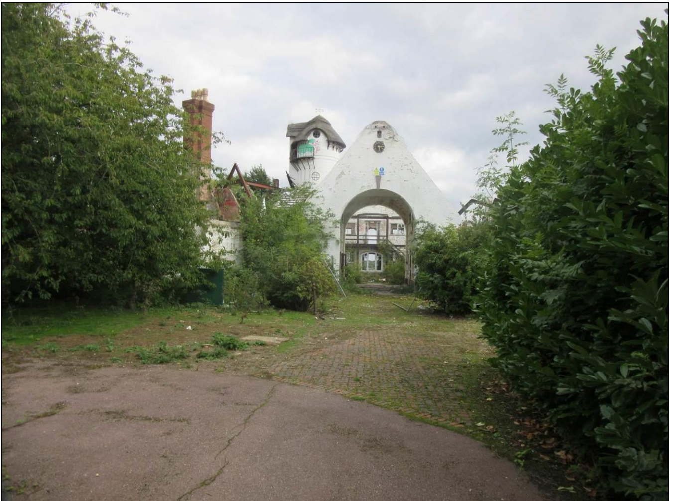
Photograph A – Looking south towards the main building.
