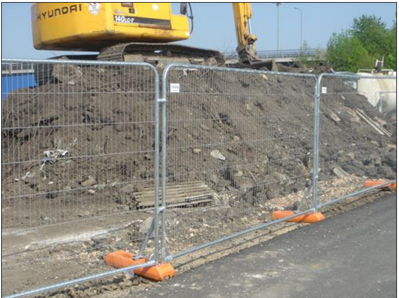
Photograph J – Example of Heras Tree Protective Fencing
