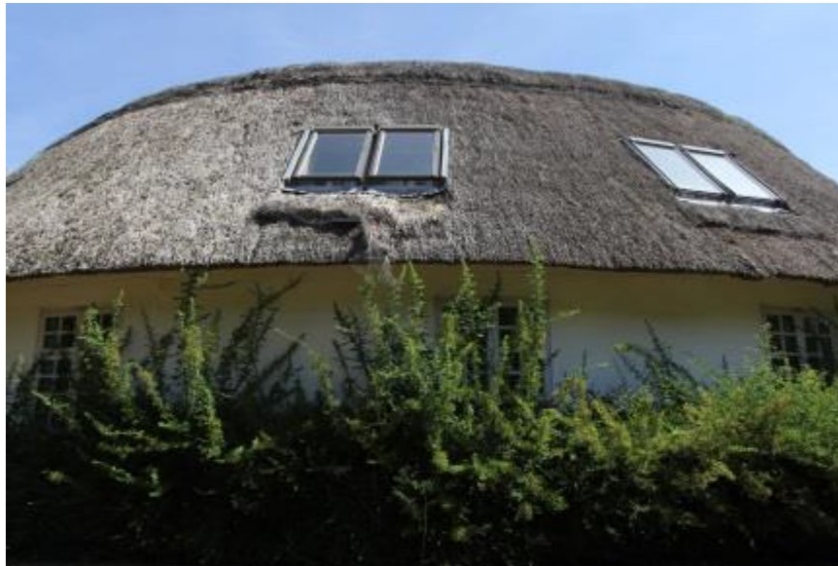
Figure 2: Section of undamaged roof (source:client)
