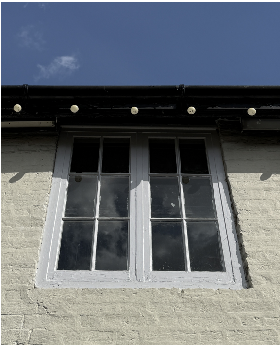
Photograph of window W1-03 (W1-01 sill is present)
