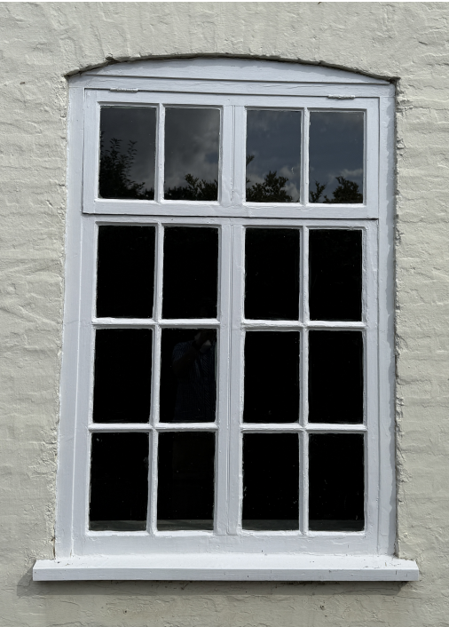
Photograph of windows WG-01, 02 & 03.
