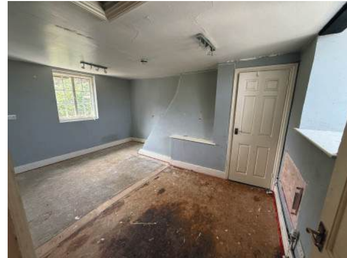
FORMER BEDROOM 3 - NOW TO BE CONVERTED TO FORM EN-SUITE BATHROOM
