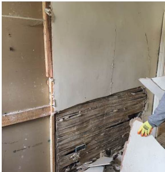
PHOTOGRAPH OF PARTITION DURING OPENING UP WORKS
