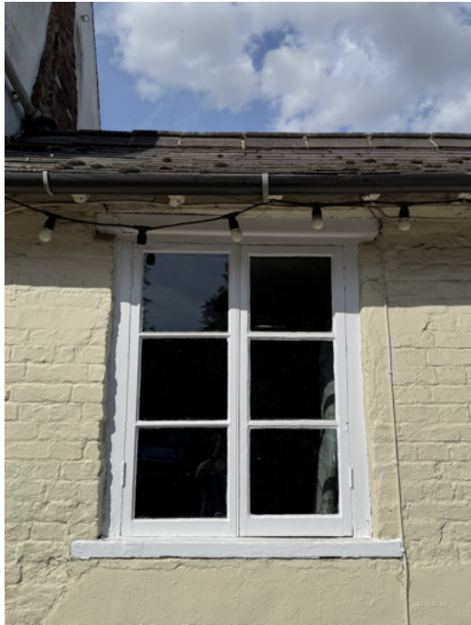
WG-06 on the (flank) Waterdell Lane elevation.
