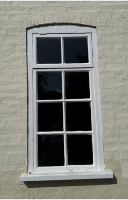
WG-05 on the (flank) Waterdell Lane elevation.
