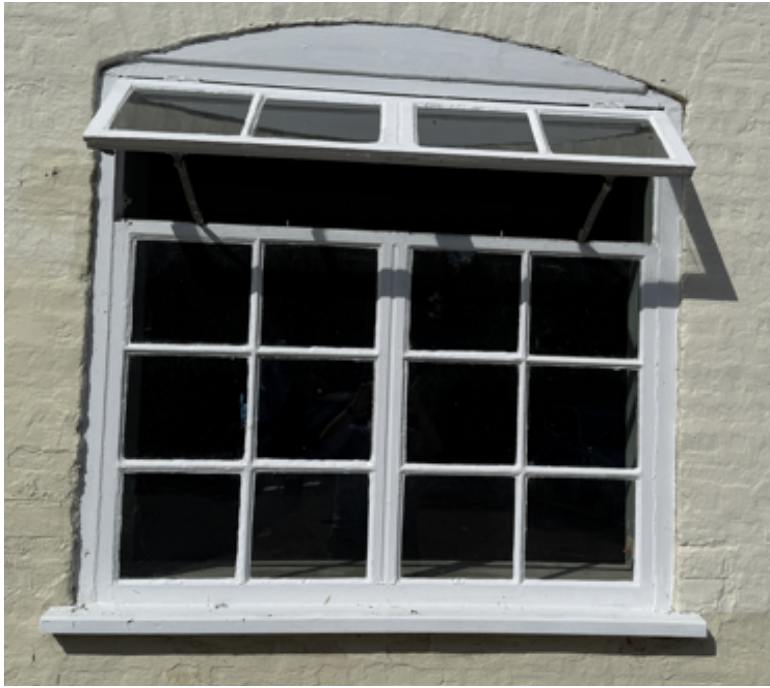
WG-04 on the (flank) Waterdell Lane elevation.
