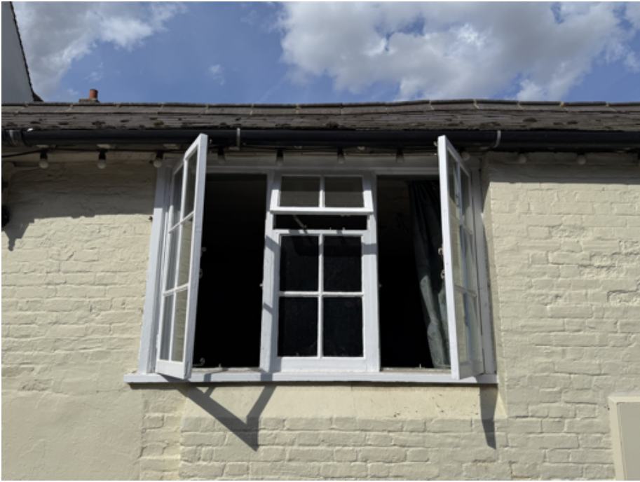
WG-07 on the (flank) Waterdell Lane elevation.
