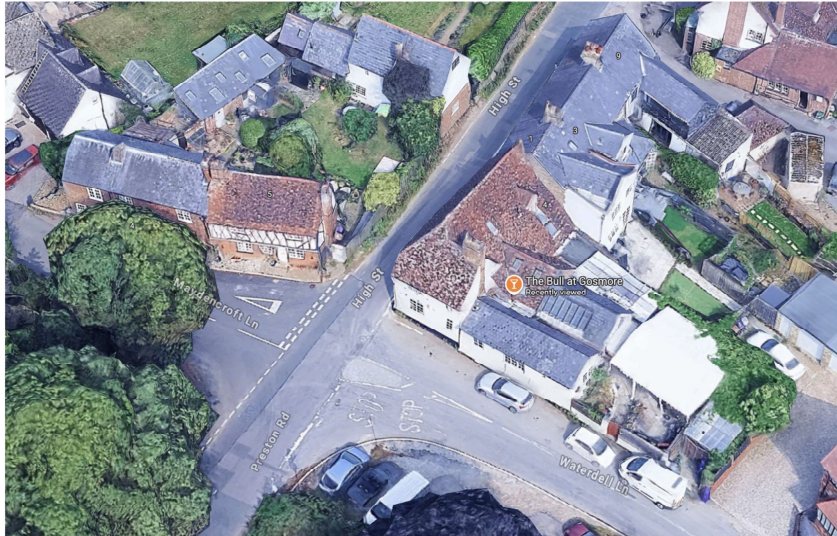
Aerial view of The Bull showing varying roof forms
