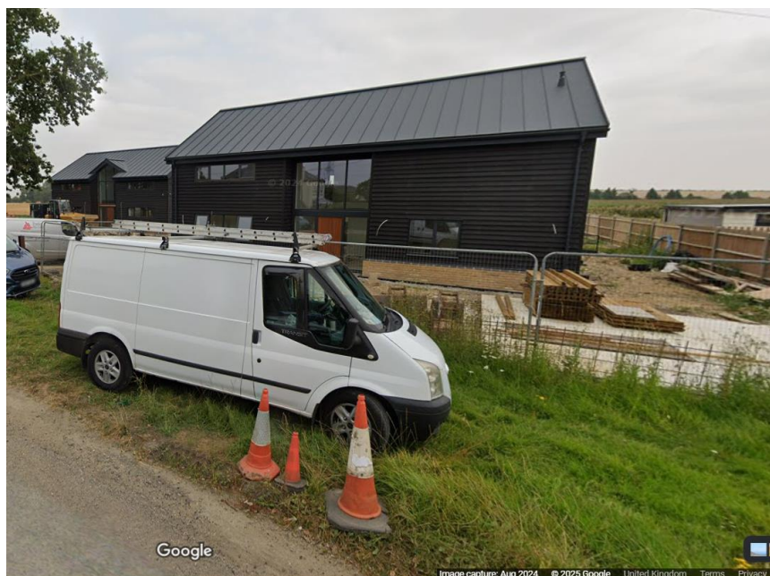
Figure 18: Image, taken from Google Maps Street View, or two houses across Hinxworth Road from the site subject to this application
