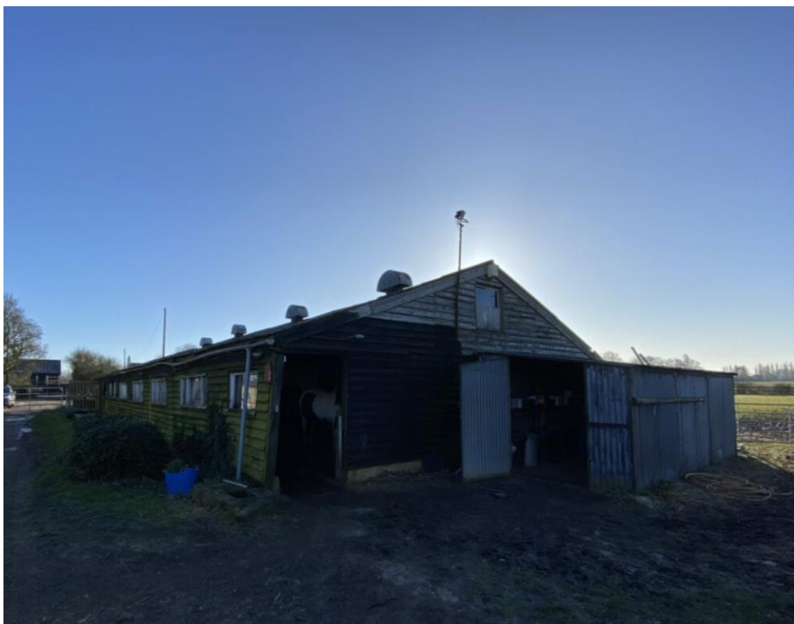
Photo 1 – Smaller Stable, West and Northern Elevations
