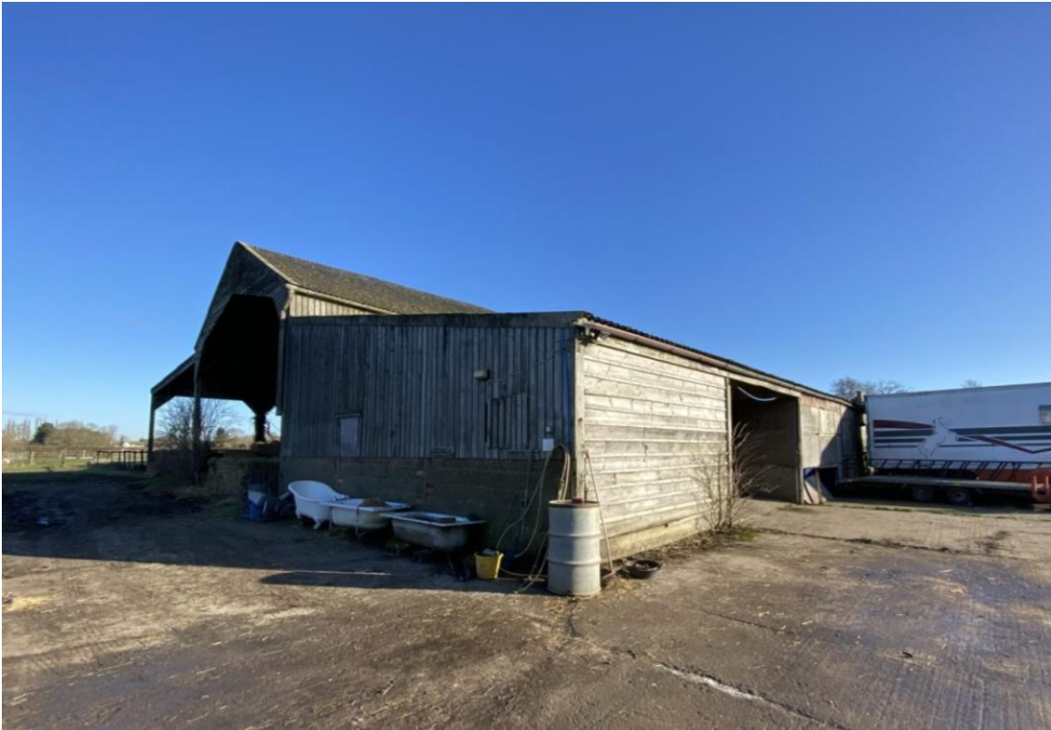
Photo 2 – Larger Stable, South and Western elevations
