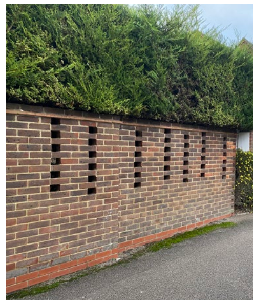
HIGH BRICK WALL WITH DETAILING
