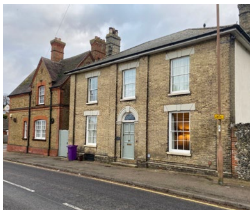
GEORGIAN BUILDING ON MARKET HILL
