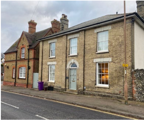
GEORGIAN BUILDING ON MARKET HILL
