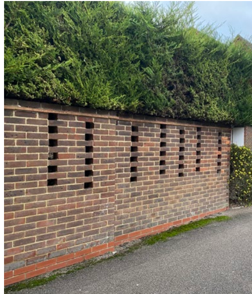
HIGH BRICK WALL WITH DETAILING
