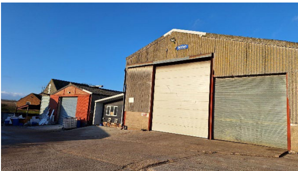
PLATE 3: VIEW SOUTH-WEST TOWARD ENTRANCE
