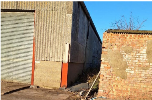
PLATE 4: VIEW NORTH-WEST BETWEEN GRAIN STORE AND BARN 1
