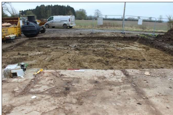
Plate 14: Stripped area, looking south
