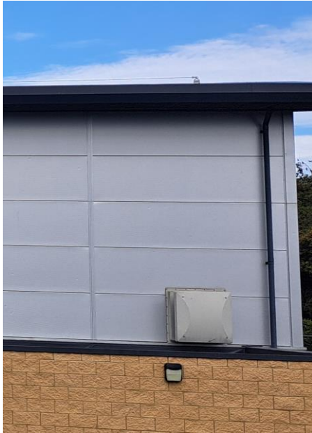
Site photo – Existing Kingspan cladding RAL 9006
