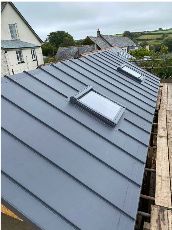
SINGLE PLY MEMBRANE STANDING SEAM ROOF
