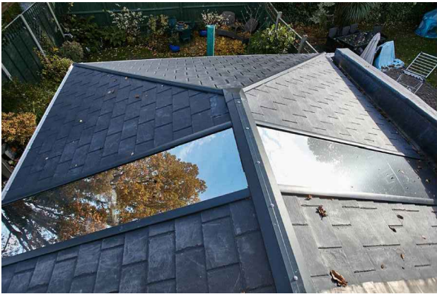
FULL LENGTH GLAZED PANELS
