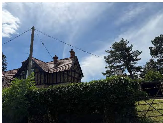
View south of Pegsdon Lodge
