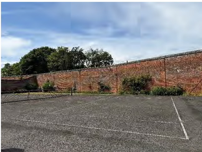
View west of tennis court
