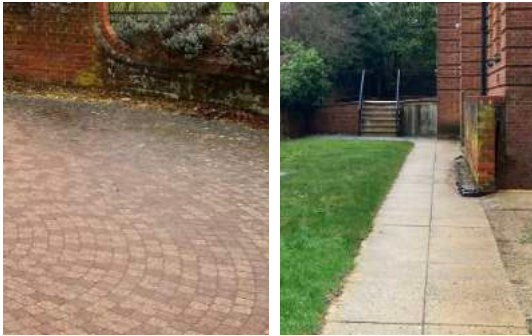
4 Existing surfaces in good condition retained and upgraded as needed
