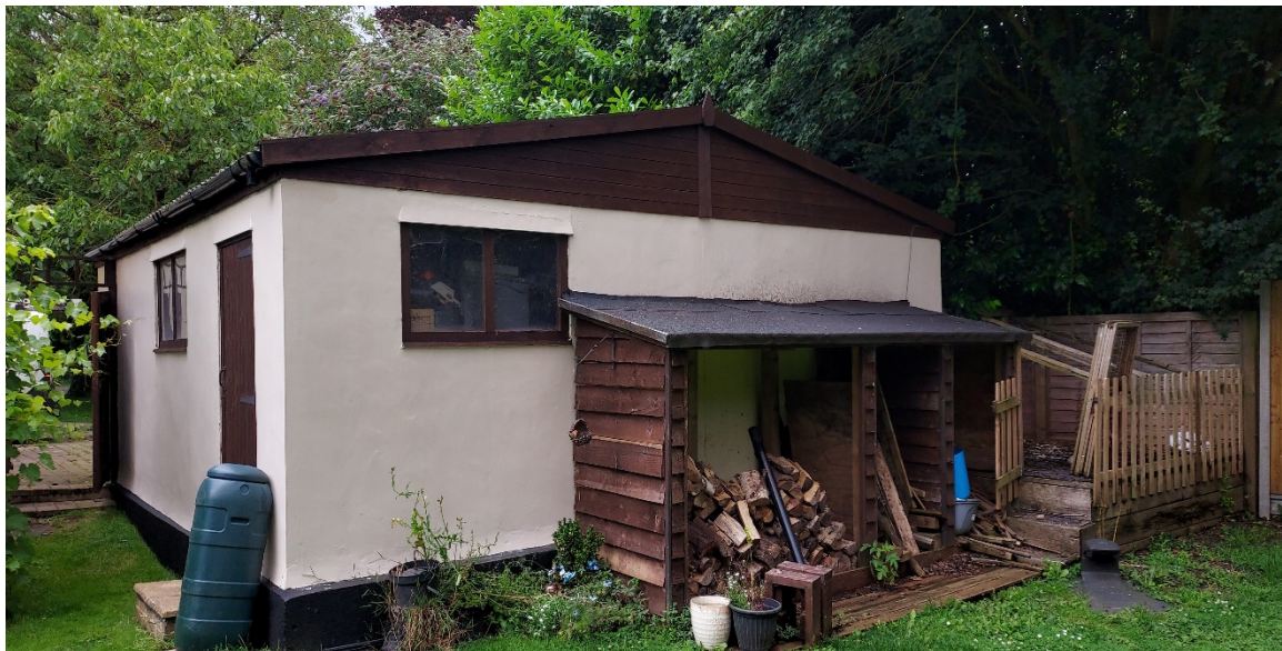
Rear elevation of Garage
