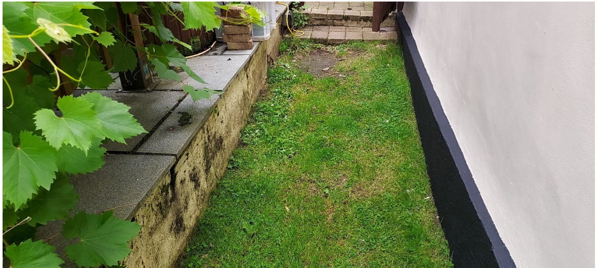
Garage adjacent rear raised patio area
