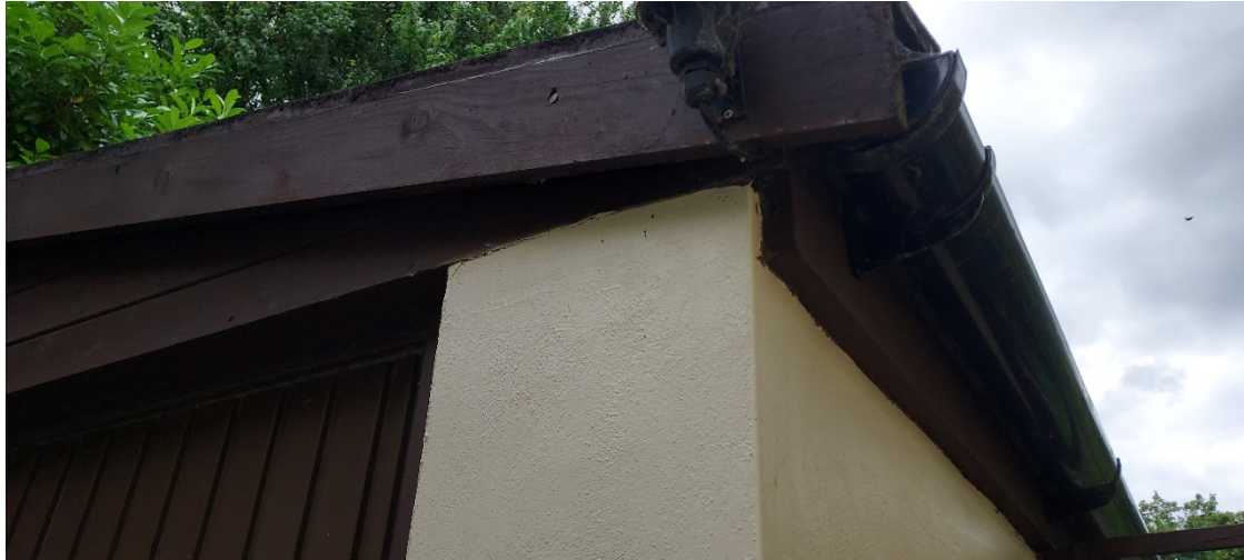
Garage front eaves detail
