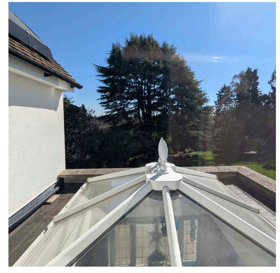
View over the existing kitchen lantern roof
