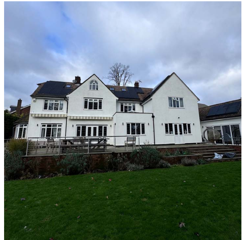
View of the existing south east elevation
