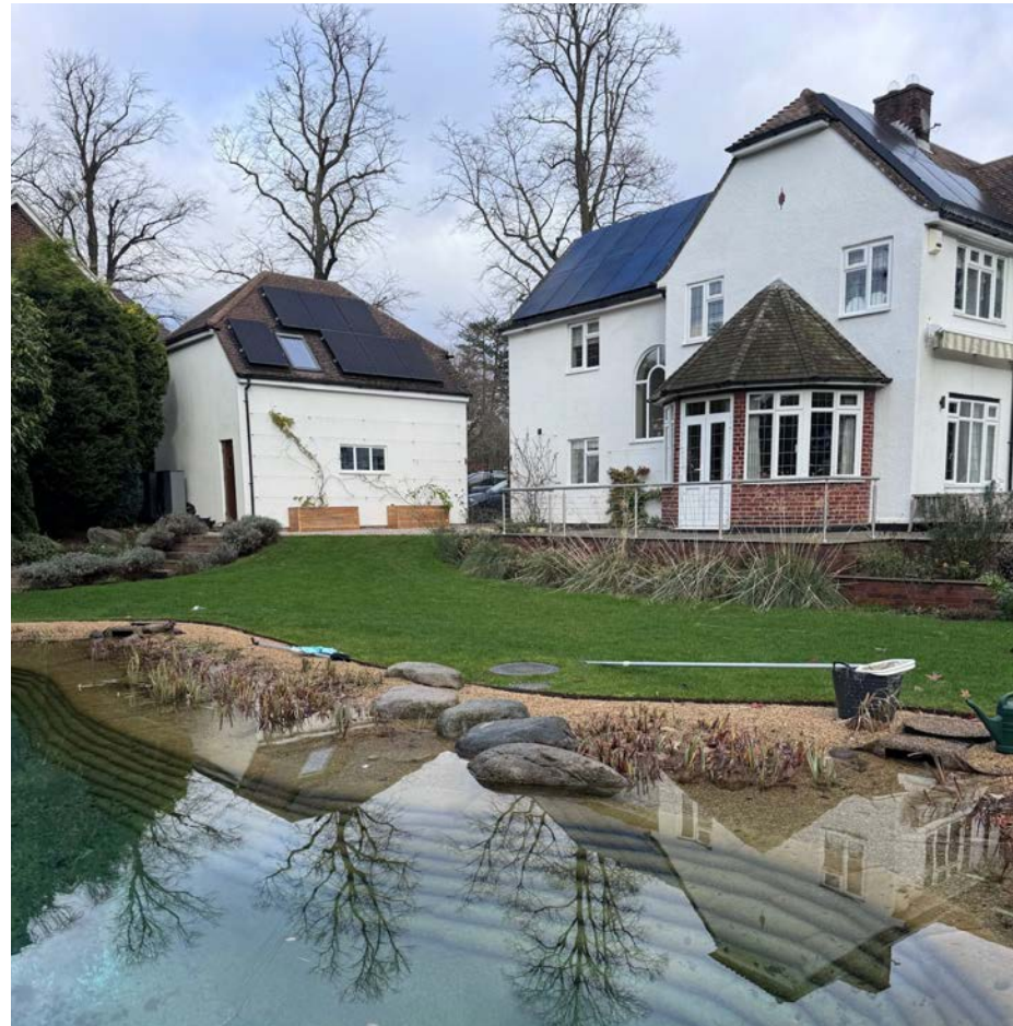
View of the existing south west elevation
