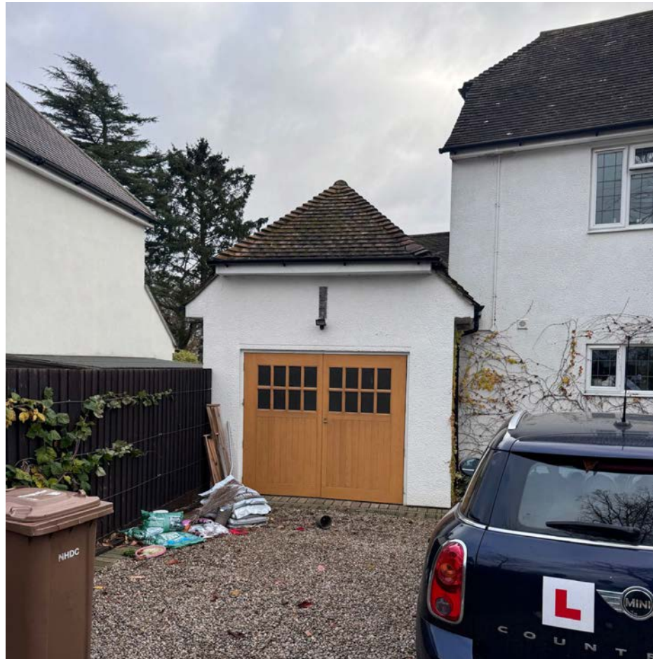
View of the existing garage
