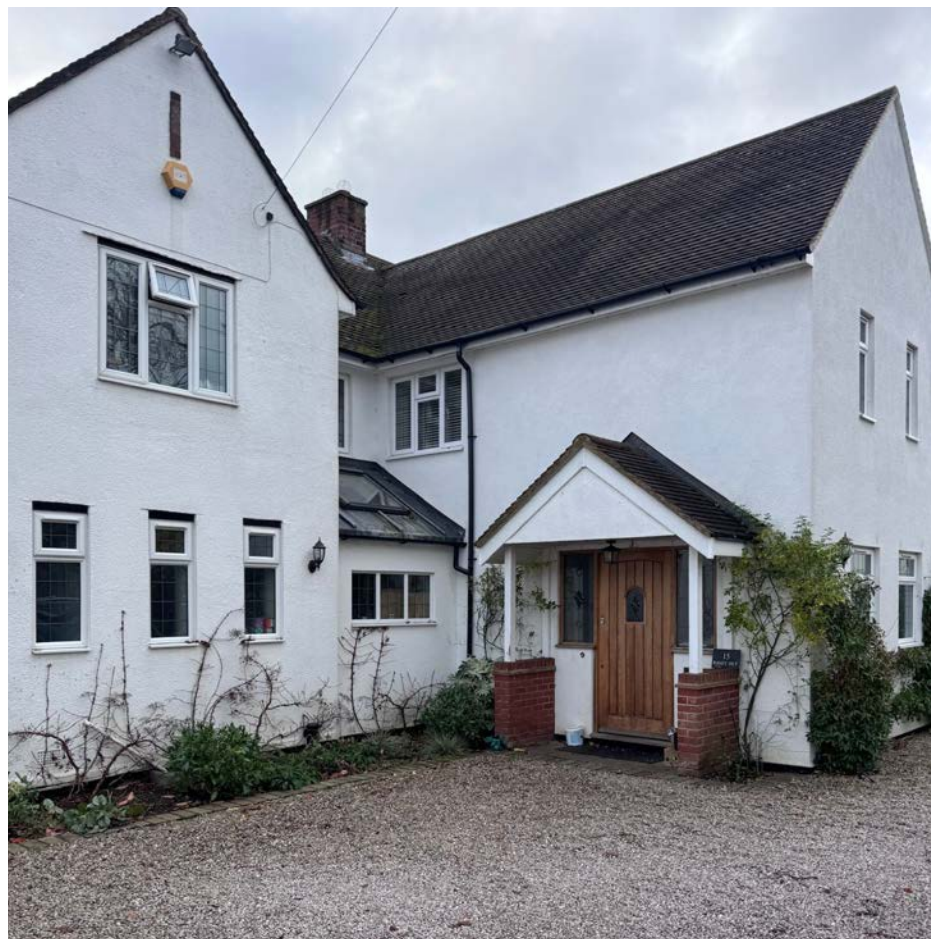
View of the front porch and entrance
