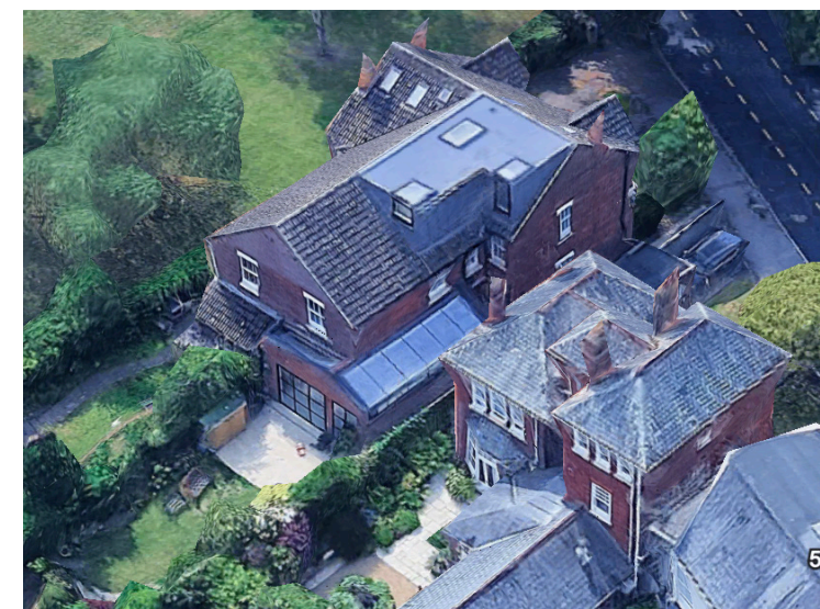
Example dormer and rear extension above, 7 The Avenue
