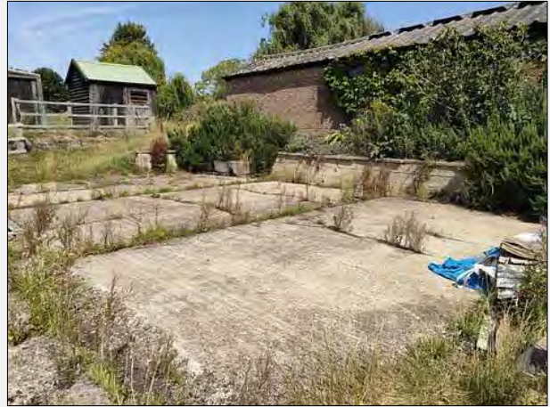
Plate 6: Northeastern external area facing neighbours outbuilding
