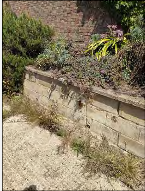
Plate 12: Northeastern external area facing neighbouring outbuilding
