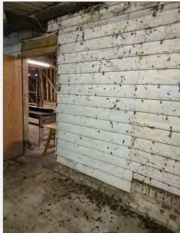
Plate 14: Internal lean-to facing barn
