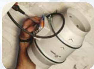
Carry out the wiring connections
