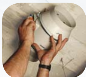
Place the impeller and motor assembly
