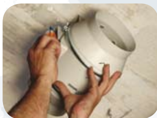
Place the impeller and motor
