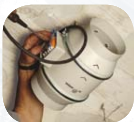
Carry out the wiring connections
