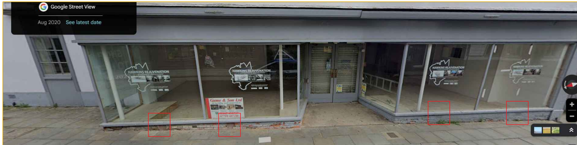
GOOGLE PHOTO OF AUGUST 2020 SHOWING AIR BRICKS
