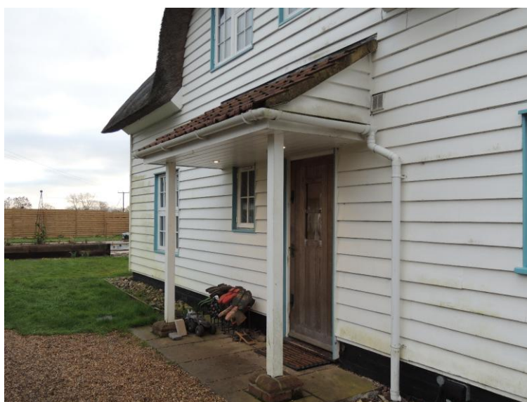
Photo 2: The porch is to be replaced
