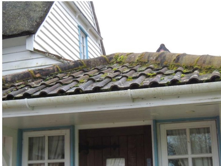
Photo 5: Note tight seal to tiles
