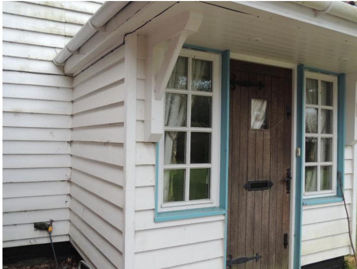
Photo 4: Showing extent of area to be removed
