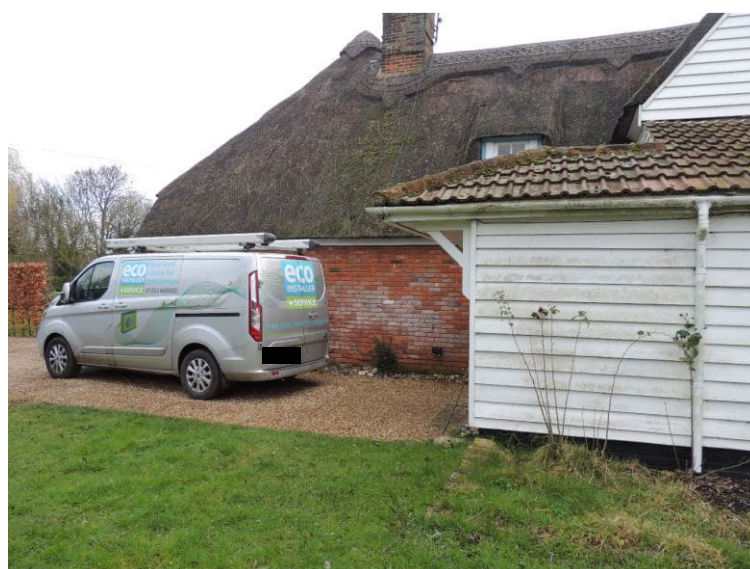
Photo 3: The short section from, and to the left of the downpipe is to be removed
