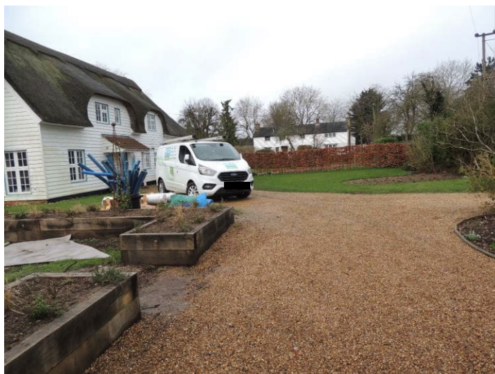
Photo 13: Showing extent of gravel to north
