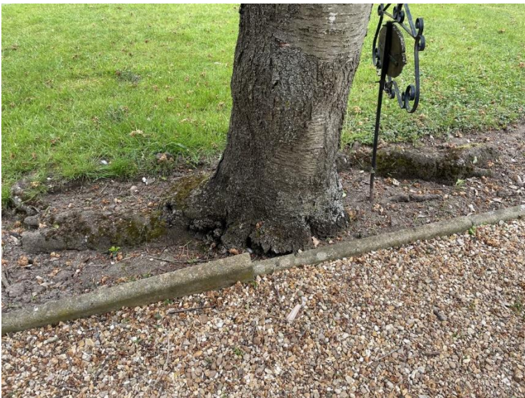
TC3 (13.05.24) Structural roots of T43 to be retained and protected with design
