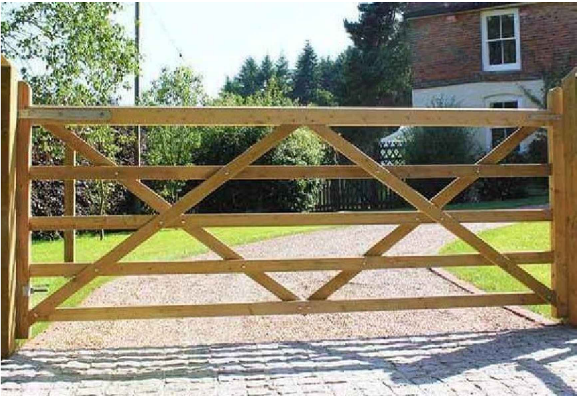
Gates all to be timber 5 bar.
