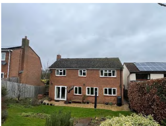
Photograph 11. Southern elevation of B1 and vegetated garden.
