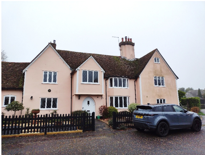
01 Front/east farmhouse elevation onto Westbury Farm Close, nos 3 & 5.
