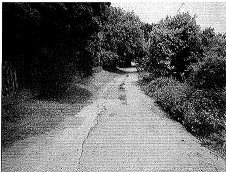
Photo 1: Photograph showing width of proposed access route and lack of adequate verge space.
