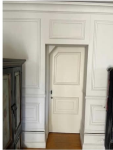
Figure 4.134: Showing the doorway from the western bedroom into the bathroom at first floor level within the sun room.
