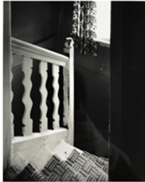
Figure 4.34: 1952-54 photograph showing the historic split balusters and newel post in the stair wing. (Source: Historic England Archives, Reference: 8892/06154).
