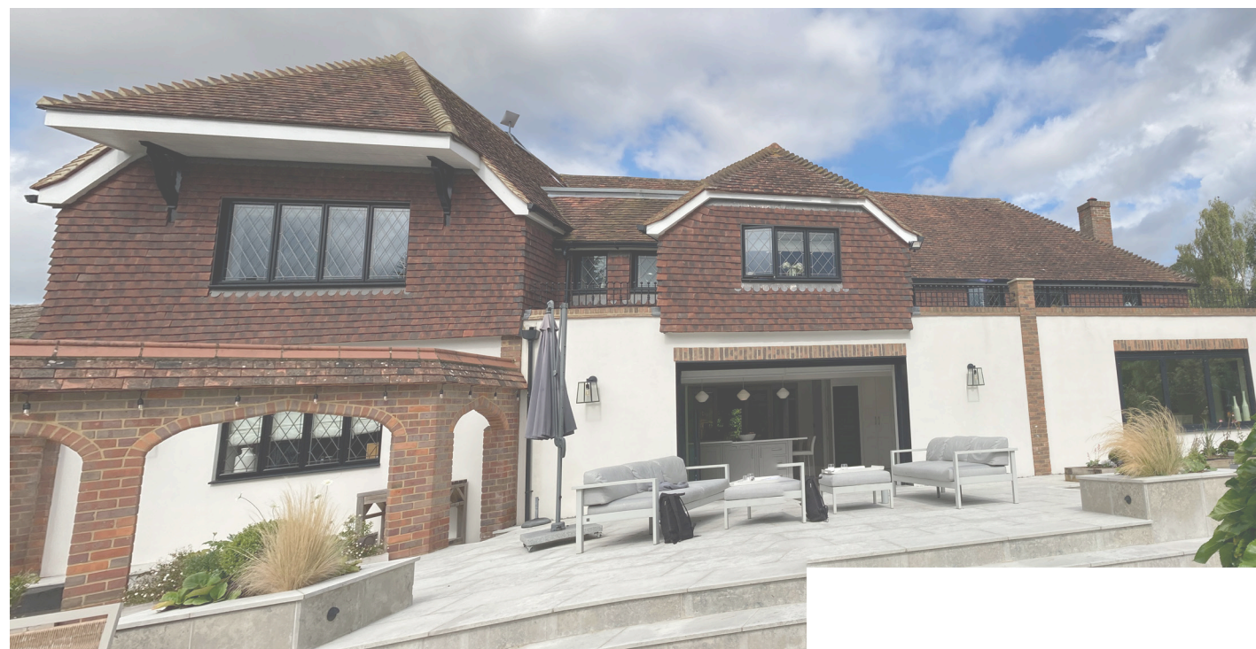
Existing rear of house
