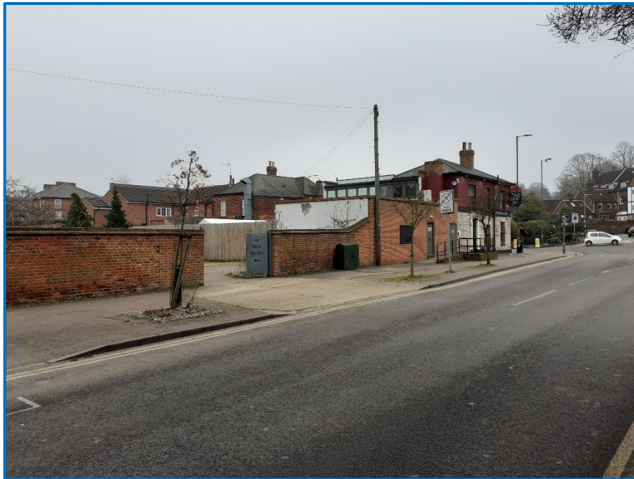
Figure 5 – View towards the site and public house from Verulam Road
