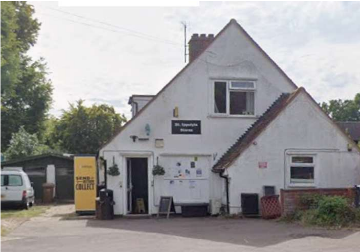
CENTRAL STORE AT WATERDELL STREET
