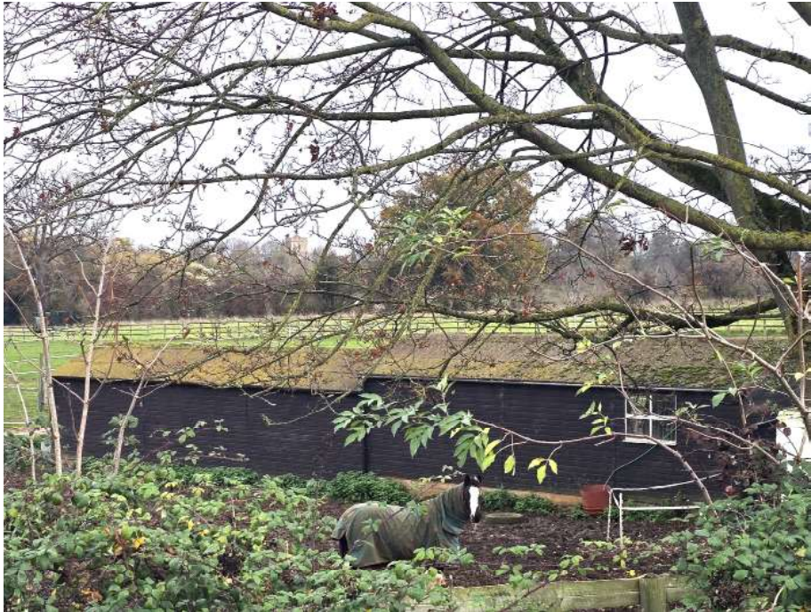
EXISTING STABLES - DARK TIMBER
