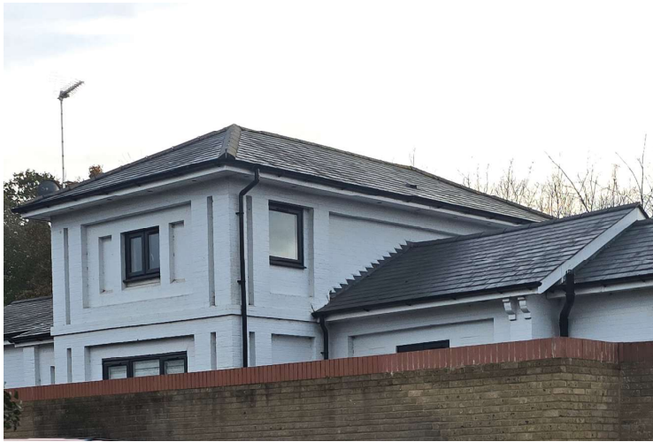
'THE FLINT HOUSE' AT LONDON ROAD
