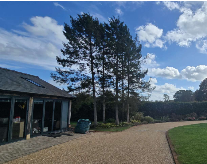
EXISTING POUND FARM OUTBUILDING & EXISTING TREES
