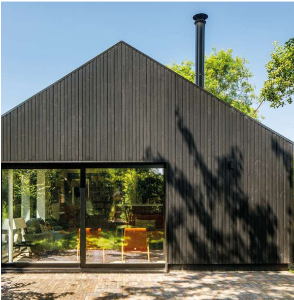
EXAMPLES OF DARK TIMBER CLADDING AND LOW EAVES
