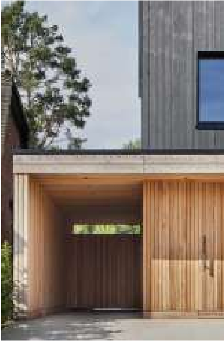
EXAMPLES OF TWO TYPES OR COLOUR TONES OF TIMBER OR TIMBER COMPOSITE CLADDING TO EXPRESS OPENINGS AND ENTRANCES - ALUMINIUM FACED WINDOWS
