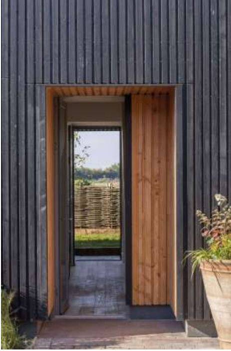
EXAMPLES OF TWO TYPES OR COLOUR TONES OF TIMBER OR TIMBER COMPOSITE CLADDING TO EXPRESS OPENINGS AND ENTRANCES - ALUMINIUM FACED WINDOWS
