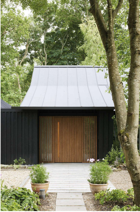
ZINC ROOF AT LONG BARN BY TAS ARCHITECTS
