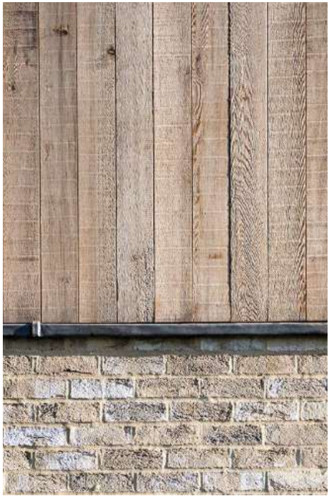
EXAMPLE OF TIMBER CLADDING WITH BRICK BELOW
