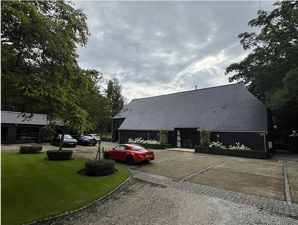
Photo 1 – Frontage of Roe Green Barn
