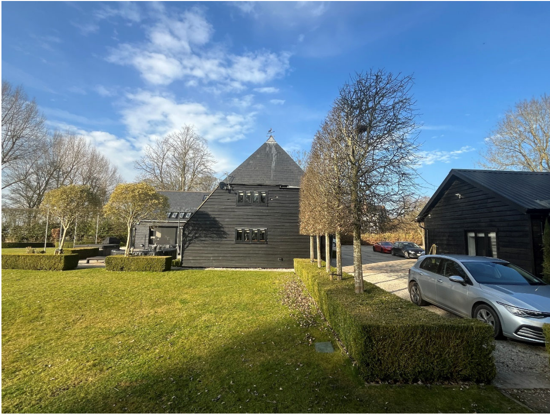
Photo 4 – Side of barn and outbuilding
