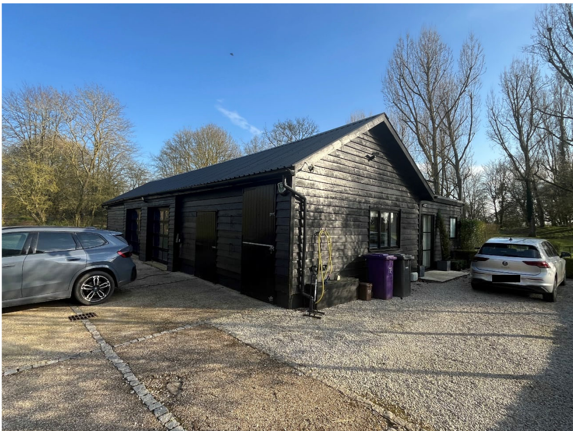
Photo 3 – Front / side rear of outbuilding
