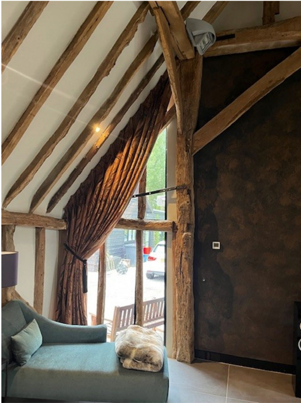
Photos 6 and 7 – Timber framing and glazing at end of aisle within lounge
