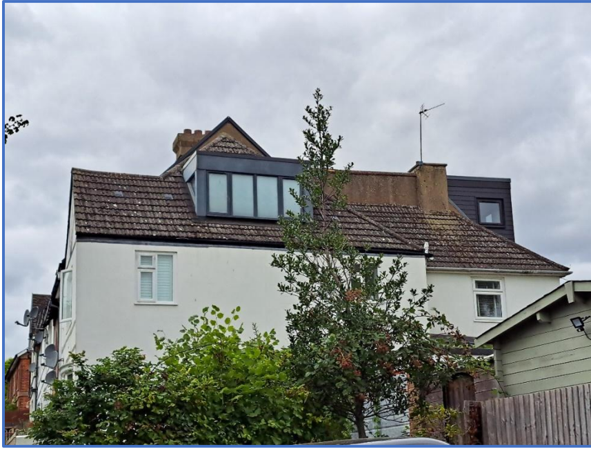
Figure 9 – View of the development from Gaping Lane (on right, with side dormer window at No. 32 to left) – materials to be changed to matching hanging tile
