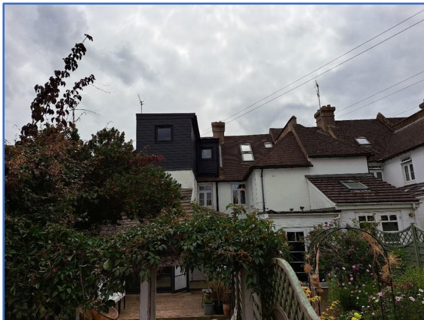
Figure 8 – View of existing rear elevations of the adjacent properties
