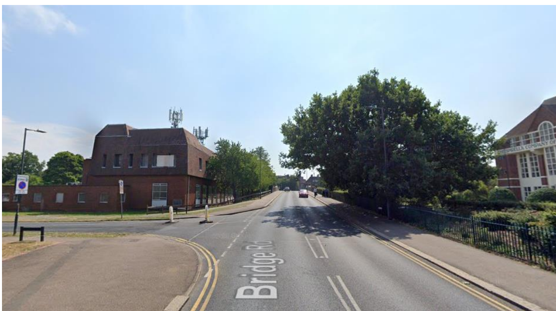
Northwestern elevation of site from Bridge Road (Google Maps)
