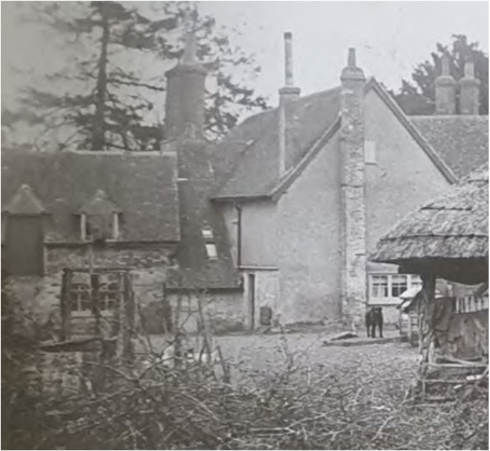
Photo 1908 facing the west end of the east-west gable range, chimney on the face of the gable no longer exists, GF window is now bigger and central. The render/brick exposed has changed over time. Hatch at loft level adjacent to chimney present.
