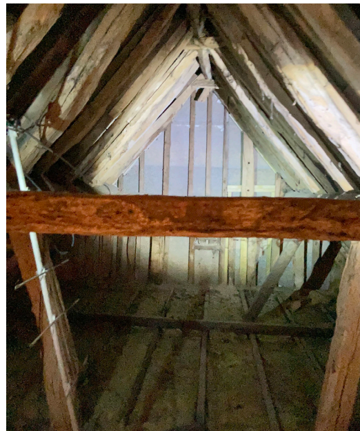
Photo of loft space over bedroom 5&6 looking north towards end gable. New breathable render carrier board visible between the end timber studs.
