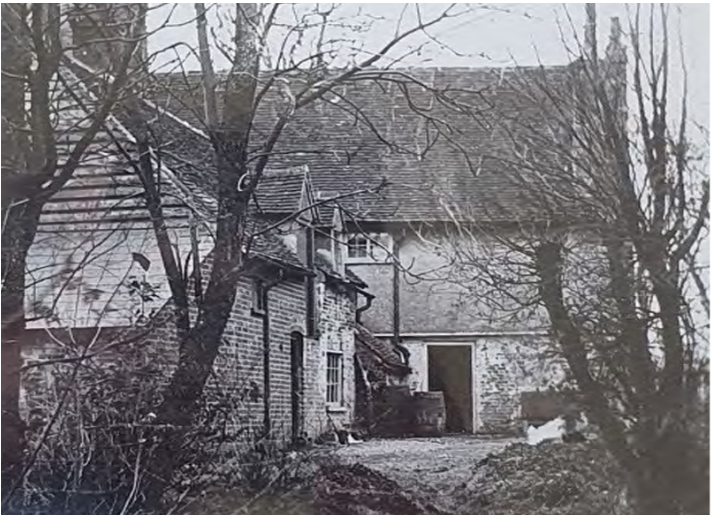
Photo 1908 facing the north side of the east-west gable range, door has since been bricked up
