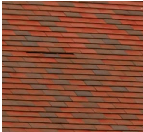
12 Example photo of tile vent
