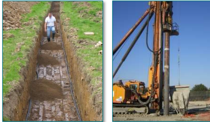
Left: Horizontal Array Trench. Right: Rig Drilling boreholes for Vertical Array
