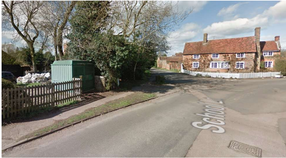
Substation location of the adjacent main road
