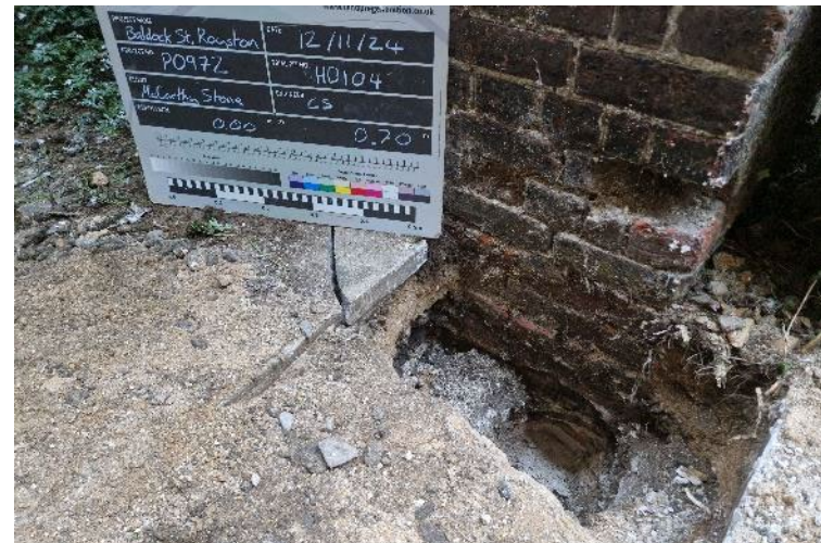
PLATE 12 – Trial Pit Excavation – HD104
