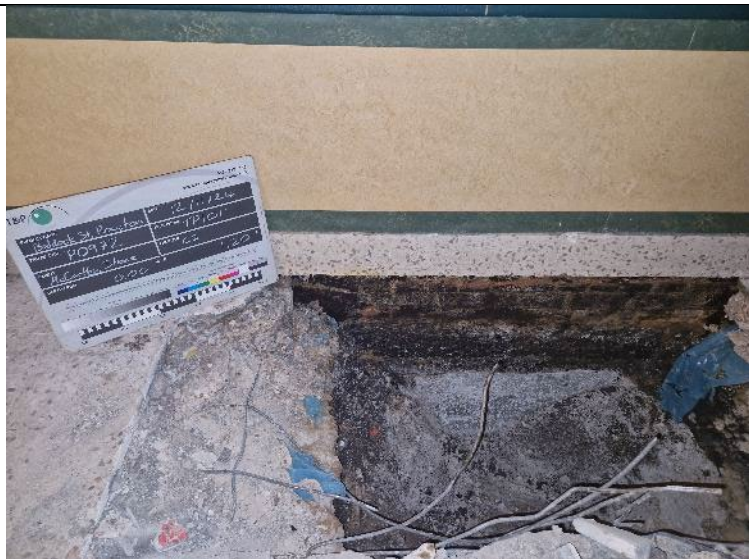
PLATE 07 – Trial Pit Excavation – TP101.
