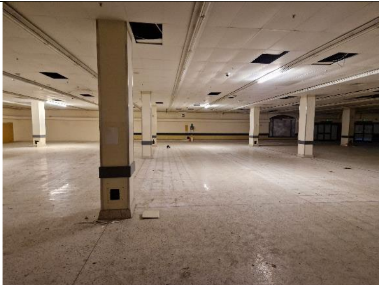
PLATE 03 – Site overview – inside the building.
