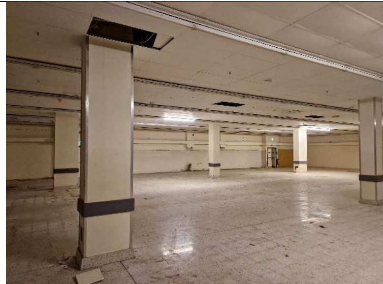
PLATE 04 – Site overview – inside the building
