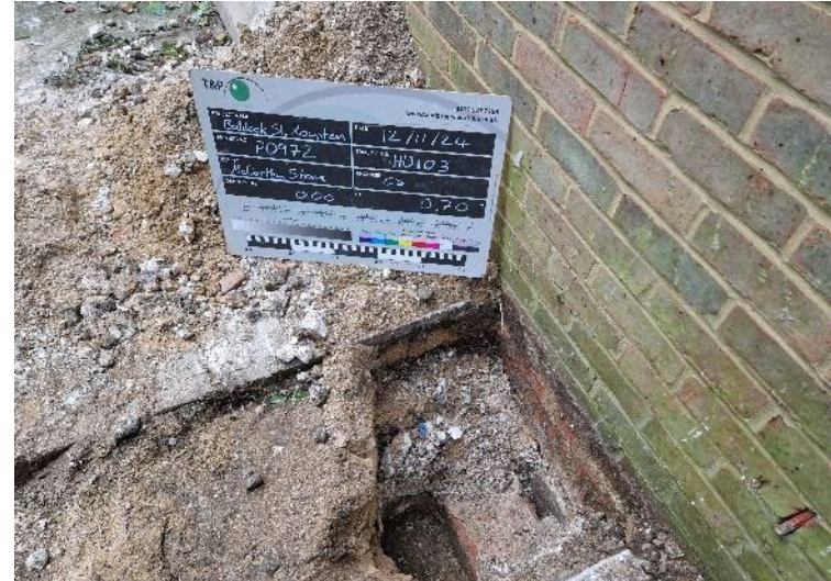
PLATE 10 – Trial Pit Excavation – HD103
