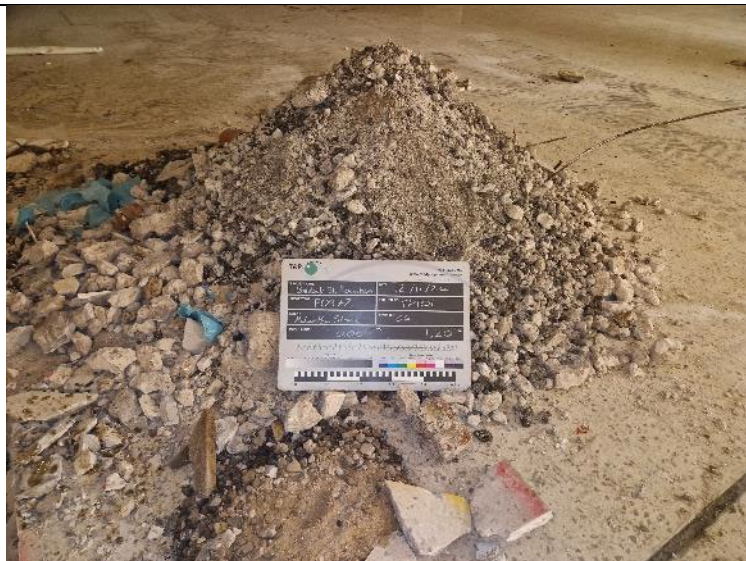
PLATE 15 – Trial Pit Spoil – TP101.
