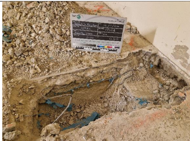
PLATE 08 – Trial Pit Excavation – TP102
