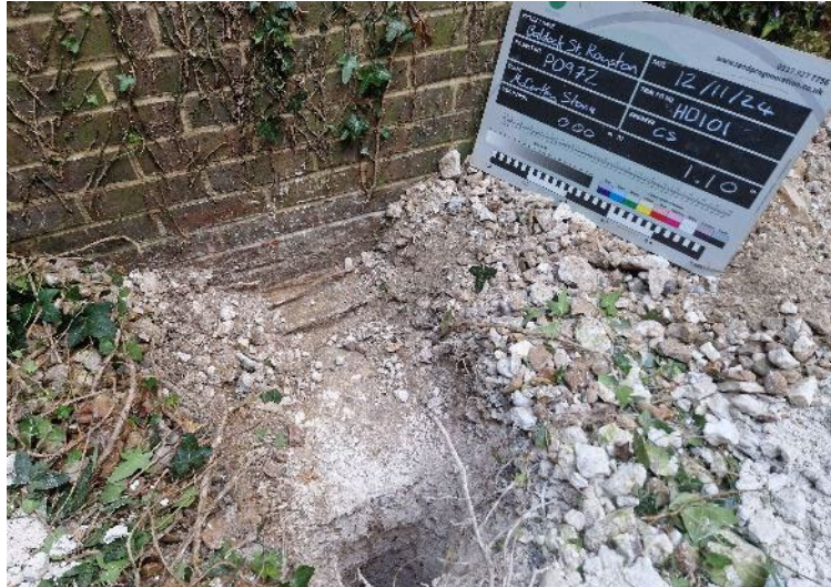
PLATE 09 – Trial Pit Excavation – HD101.
