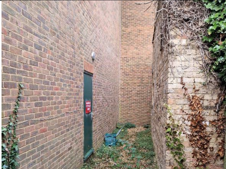
PLATE 05 – Side of the site overview.
