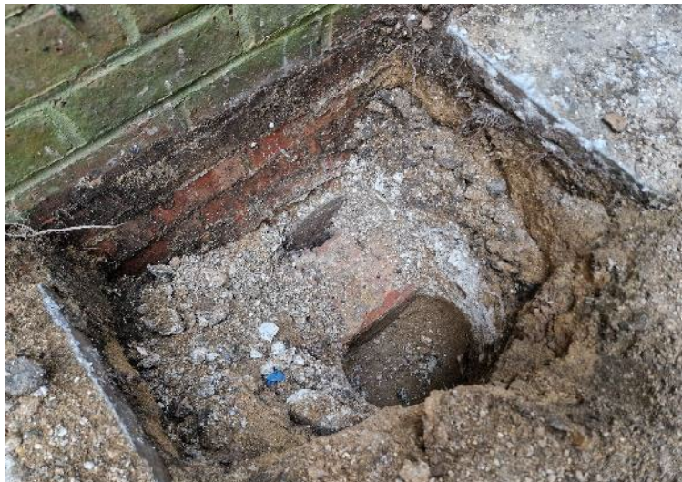
PLATE 11 – Trial Pit Excavation – HD103
