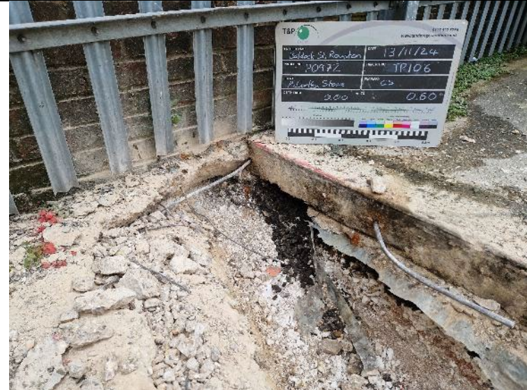
PLATE 14 – Trial Pit Excavation – TP106.
