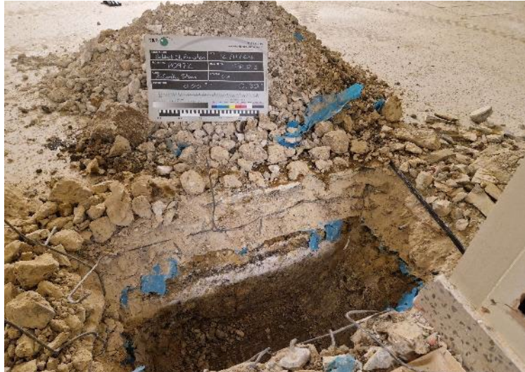
PLATE 13 – Trial Pit Excavation – TP103
