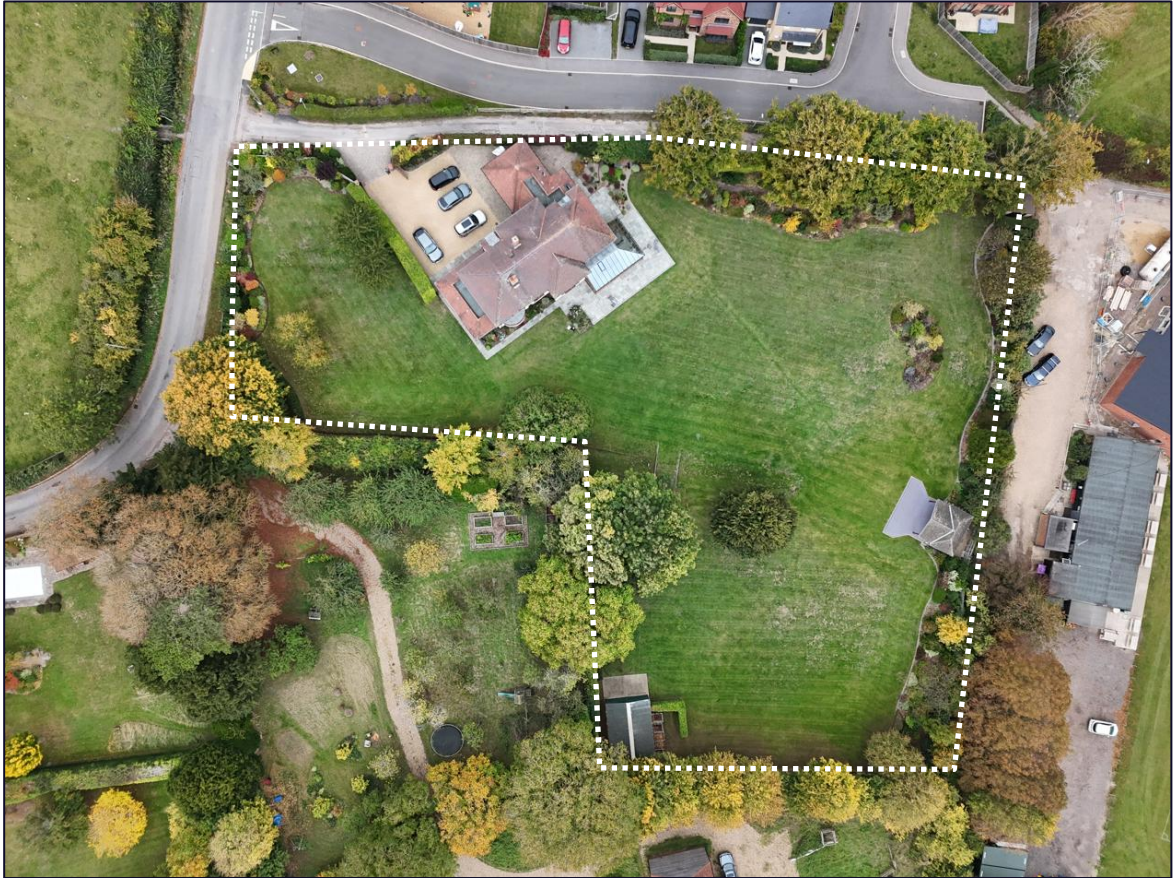
Plate 1: Aerial view of the Site in October 2025, with the property boundary of No. 19 dotted in white; North is to the top
