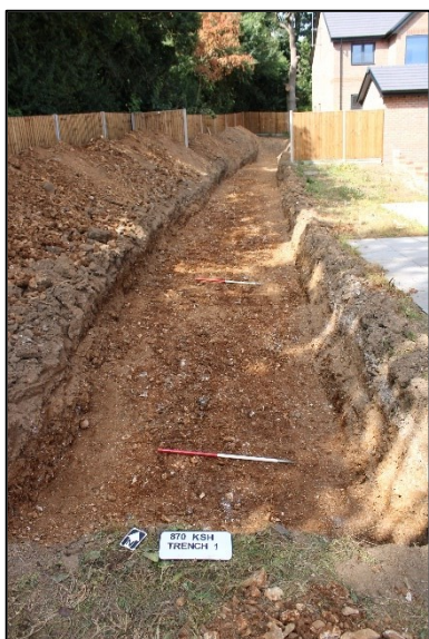
Plate 1: Trench 1, looking NE
