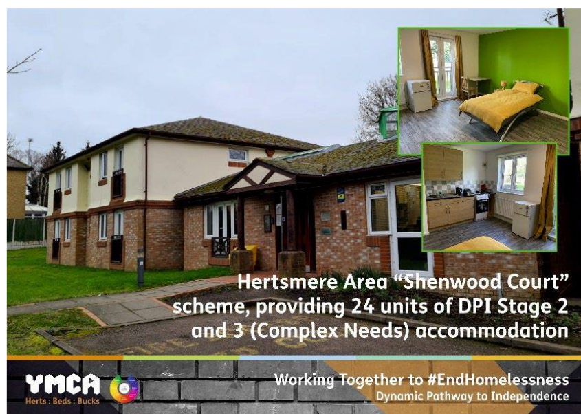
Figure 4: Shenwood Court, Borehamwood
