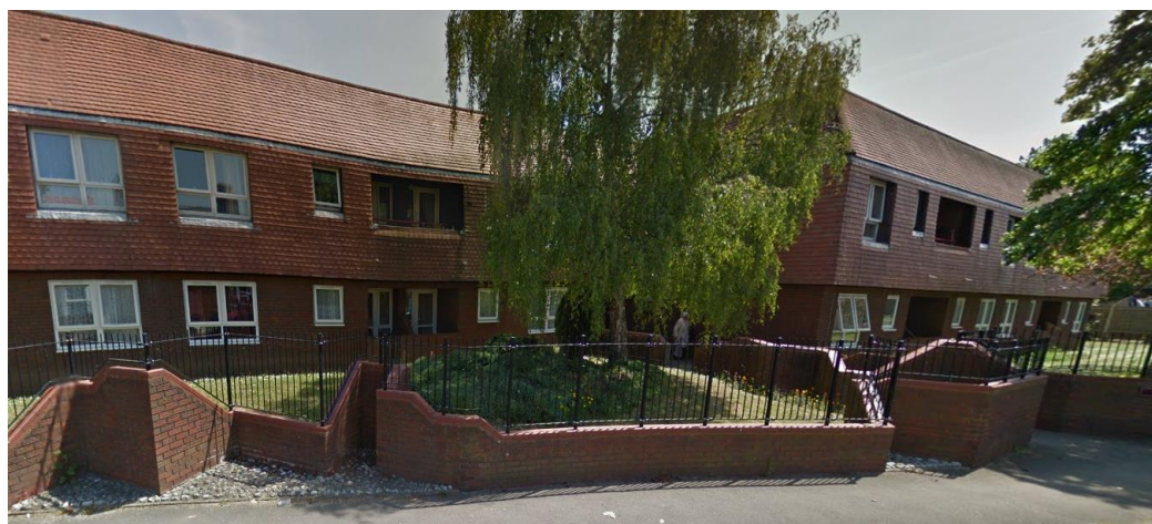
Figure 2: Andersons House, viewed from Florence Street
