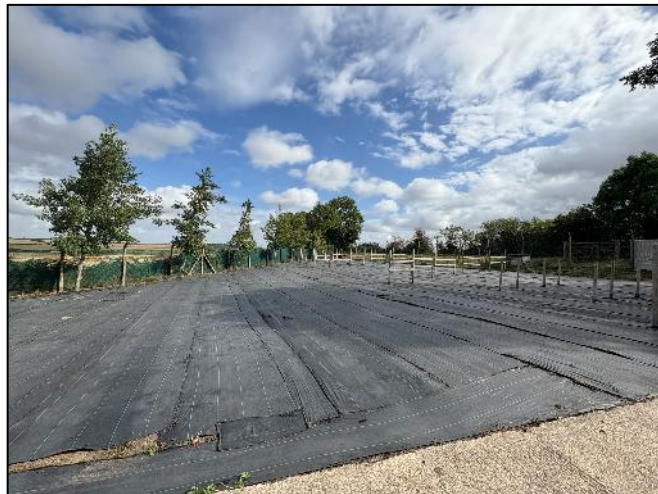
Photograph 2 Artificial unsealed unvegetated area in centre of site, with small trees along north-western boundary
