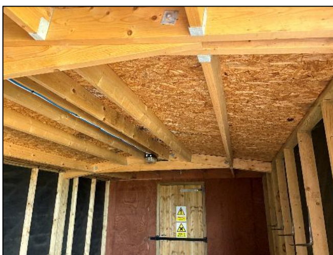
Photograph 5 Interior of shed
