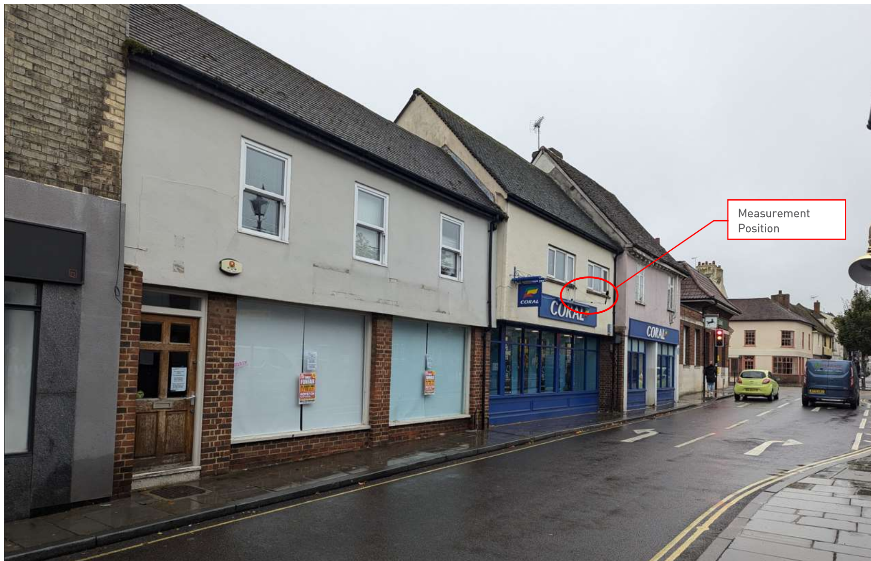
4 Kneesworth Street, Royston Site Photograph Project 13932
