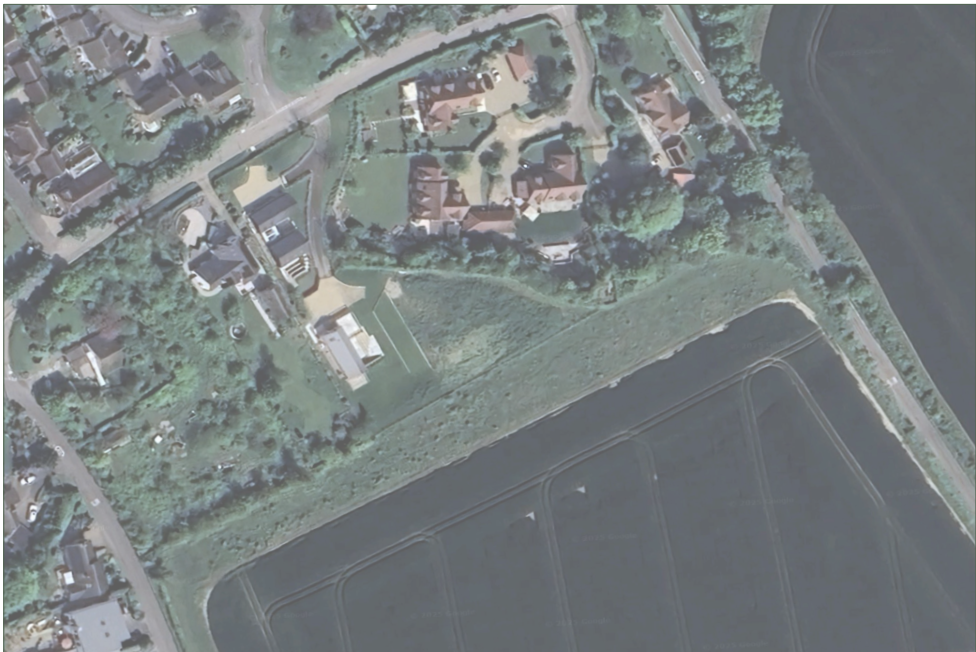
AERIAL PHOTOGRAPH SHOWING EXISTING FIELD MARGINS AND HEDGEROW NETWORK
