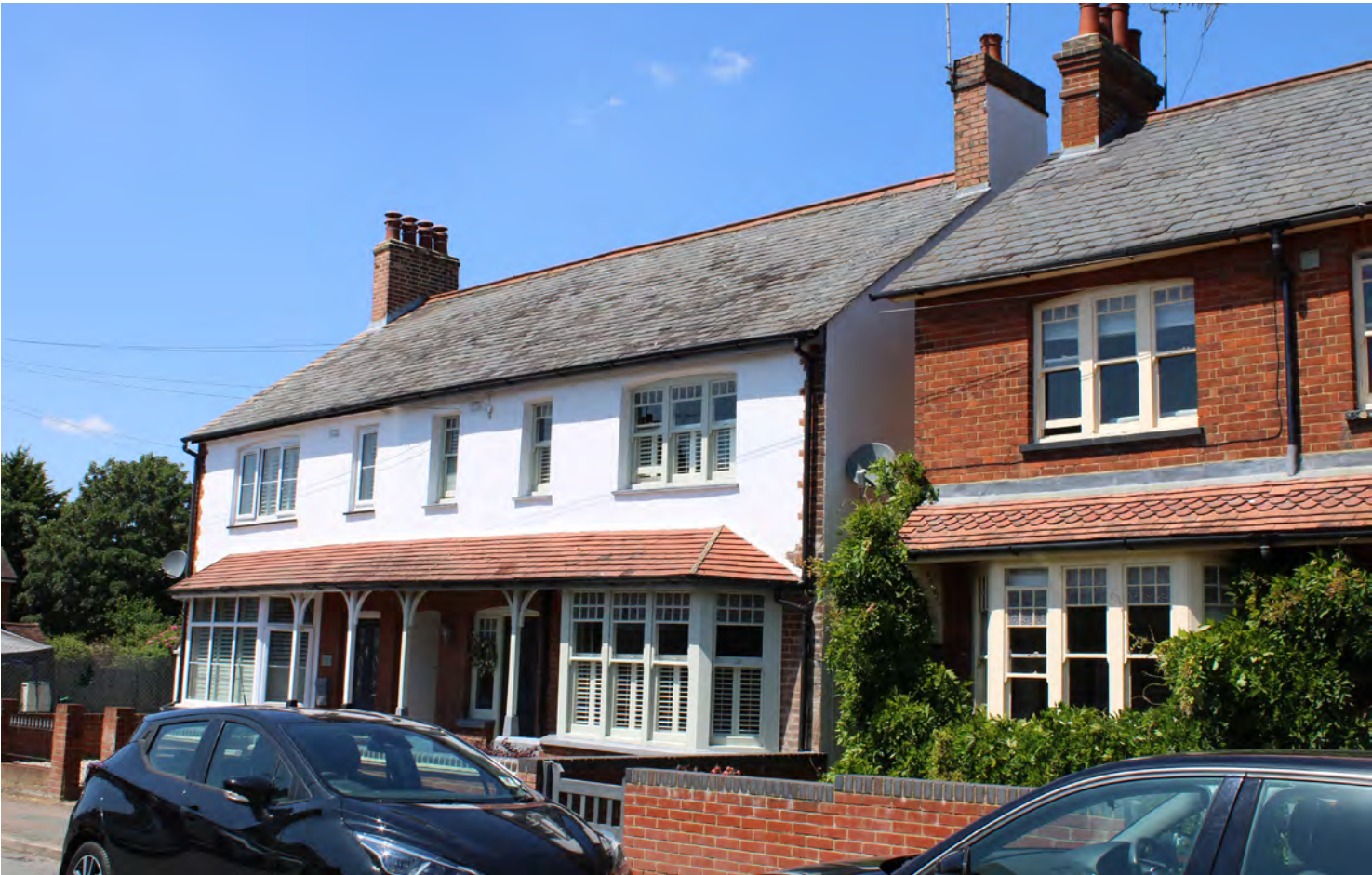
▲ There is no overriding building style in Stevenage
