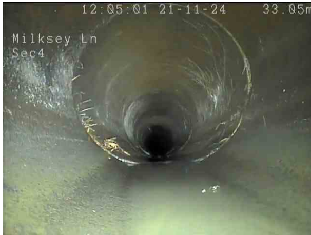
bafb911b-6cbc-4a8f-9351-8adddeb6f59d.png, 00:02:38, 33.50 m Roots, fine at joint
