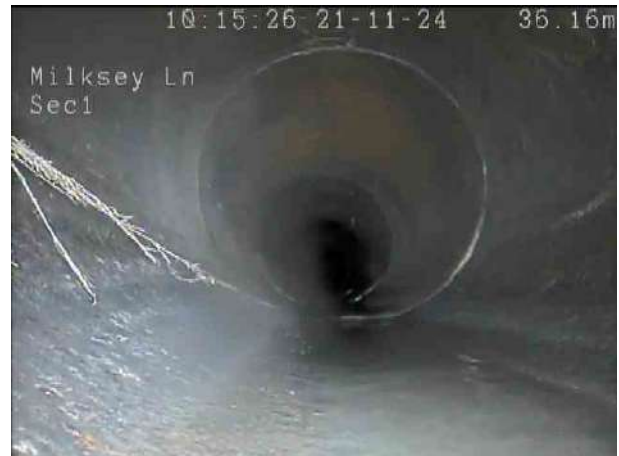
eb8eaf-11ce-49ac-99d1-1b747c865bb6.png, 00:03:41, 36.60 m Roots, fine at joint, finish
