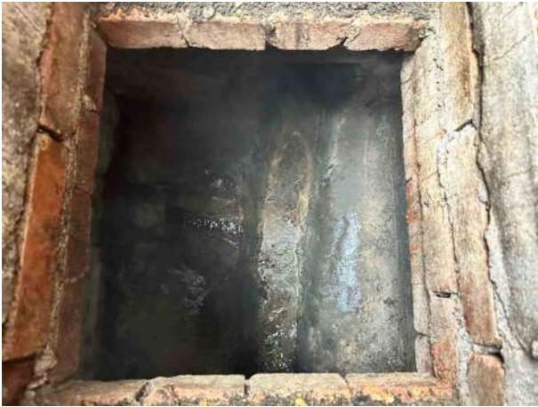
SW2.JPG, 00:00:00, 0.00 m Start node, inspection chamber, reference: SW2
