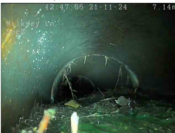
eb2e7dfa-f1ef-47fd-8f0b-1463f61647f4.png, 00:01:04, 7.10 m Roots, mass at joint, 60% cross-sectional area loss, change
