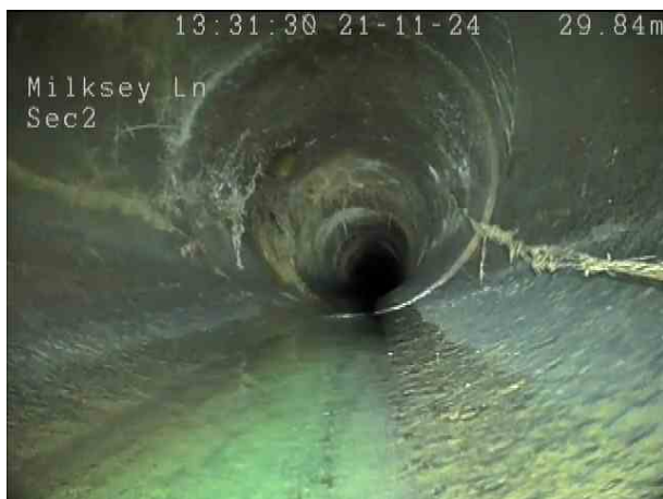
22677a1c-9702-415a-b762-6022f4cc53ea.png, 00:02:26, 30.30 m Roots, fine at joint
