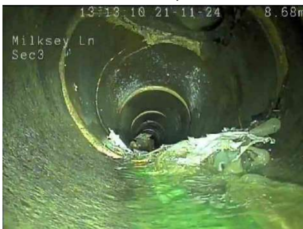
a74bc132-76af-4b72-b59a-9b0d10c1e1bd.png, 00:01:10, 8.90 m Roots, mass at joint, 10% cross-sectional area loss
