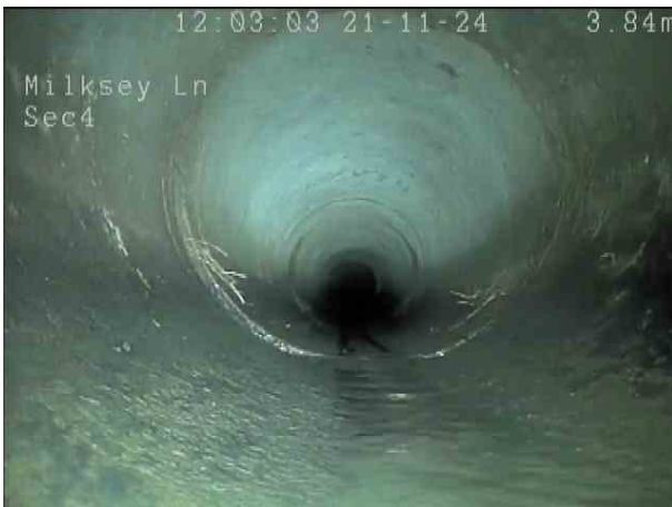
16363fe1-2ee0-4494-bdf9-0540b0de48e2.png, 00:00:40, 4.30 m Roots, fine at joint
