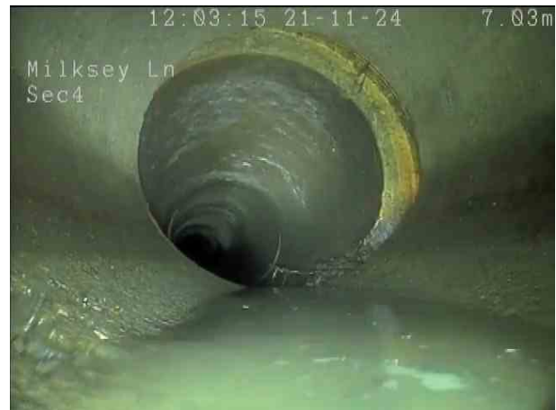
901fc6c2-b364-4fae-8fd9-338f3b128fc0.png, 00:00:52, 7.50 m Line deviates left
