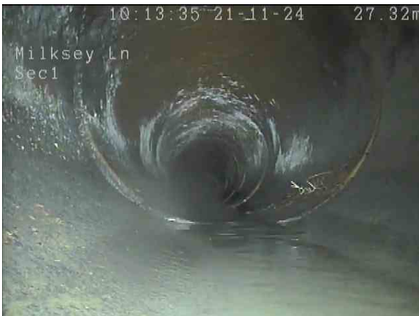
29270812-47d4-47e3-94d8-0189b74d66e6.png, 00:01:50, 28.00 m Roots, fine at joint
