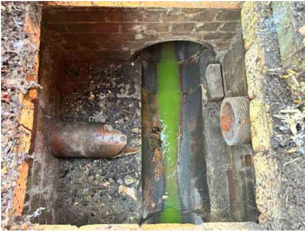
SW1.JPG, 00:00:01, 0.00 m Start node, inspection chamber, reference: SW1
