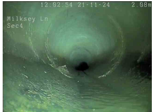
072a555f-51a2-4a4f-8c8c-0cdd0f3fb631.png, 00:00:31, 2.60 m Roots, fine at joint
