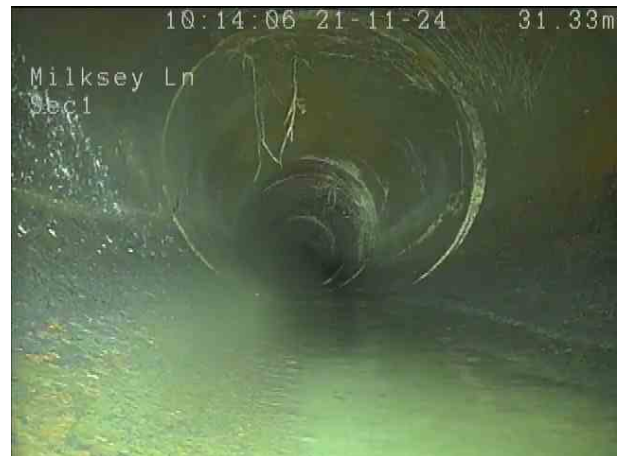
f2520338-991b-4d49-a4b7-b083027ddd3.png, 00:02:21, 32.00 m Roots, fine at joint, start
