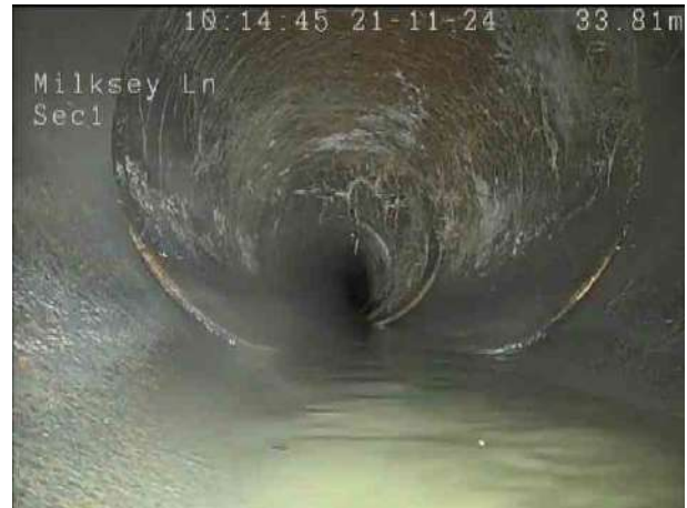
d3dc2325-8fee-4084-b3ff-8aad911865d1.png, 00:03:00, 34.00 m Roots, fine at joint, start
