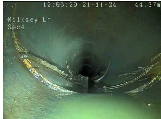
e6347e56-5449-4c1b-87a2-0c68d97f732a.png, 00:03:57, 44.50 m Roots, tap at joint, start
