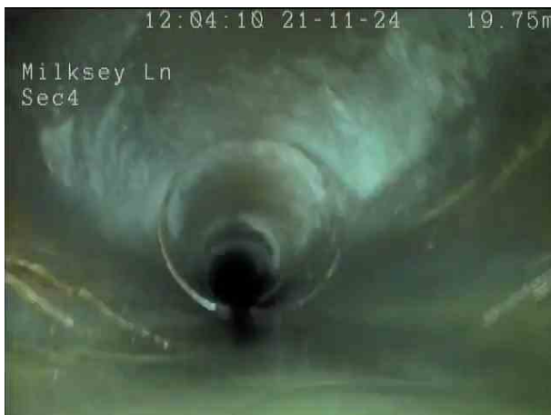
2f2d61b5-d4e9-458a-92f8-9caf123dfb0f.png, 00:01:47, 20.00 m Junction at 10 o'clock, 150mm dia
